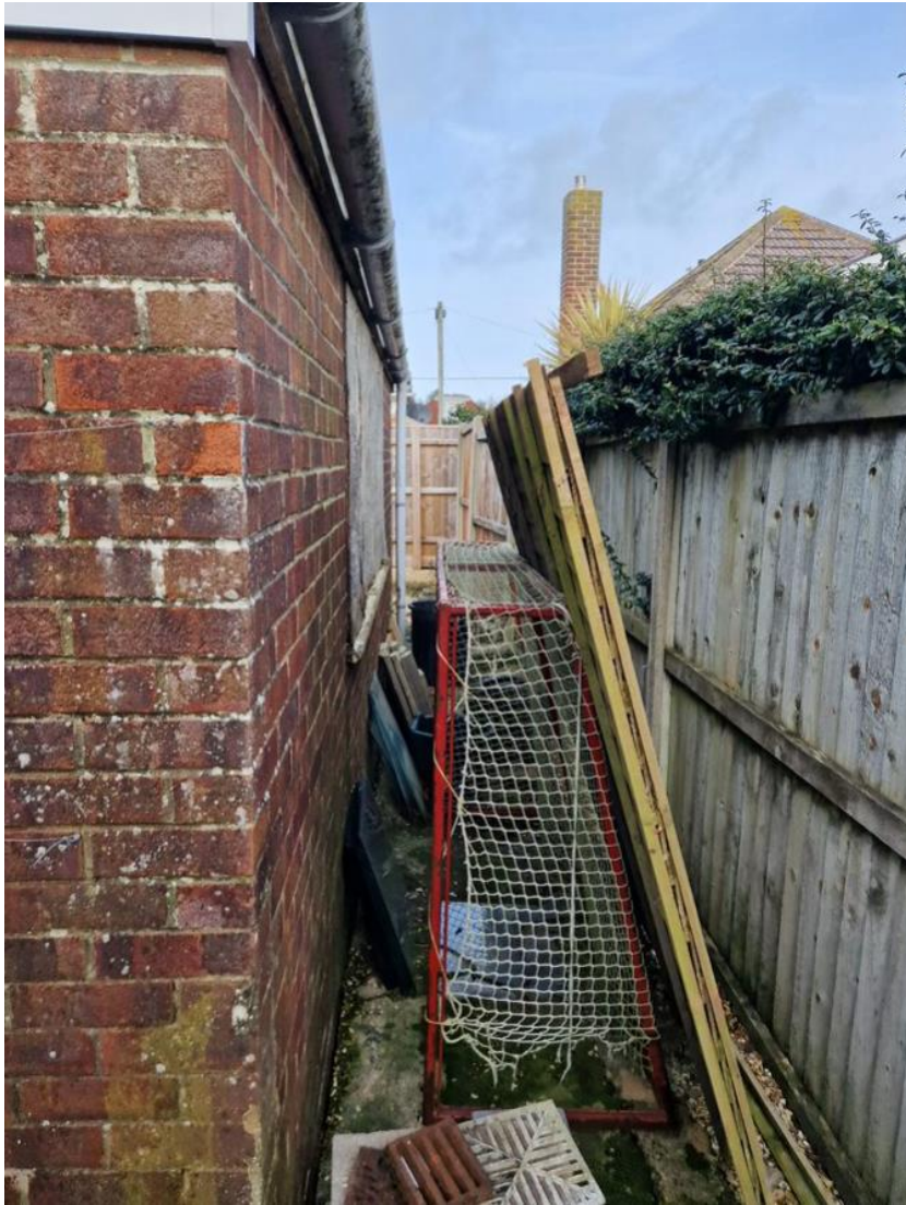
View to Rear of Garage
