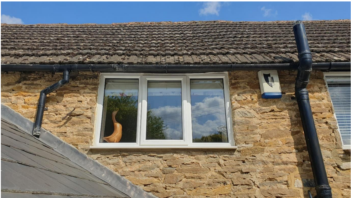
Image 10 – Existing window to No 2
