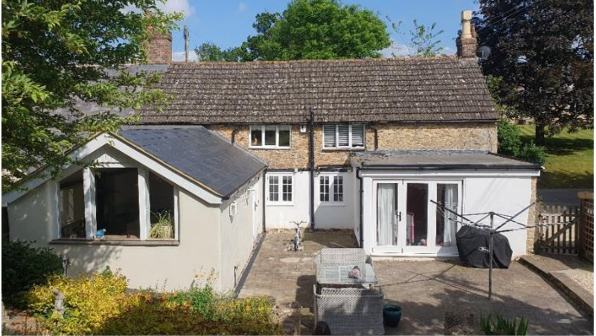
Image 9 – View of the proposed external elevation photoshopped to show the view of the rear window with the window infilled with a matching limestone. This window will be repointed as part of the main repointing. The timber lintel above the window will also be removed.
