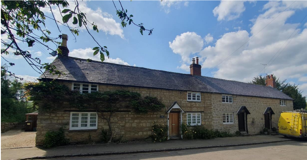
Image 1 – Front Elevation of 1-2 Main Street, Shalstone
