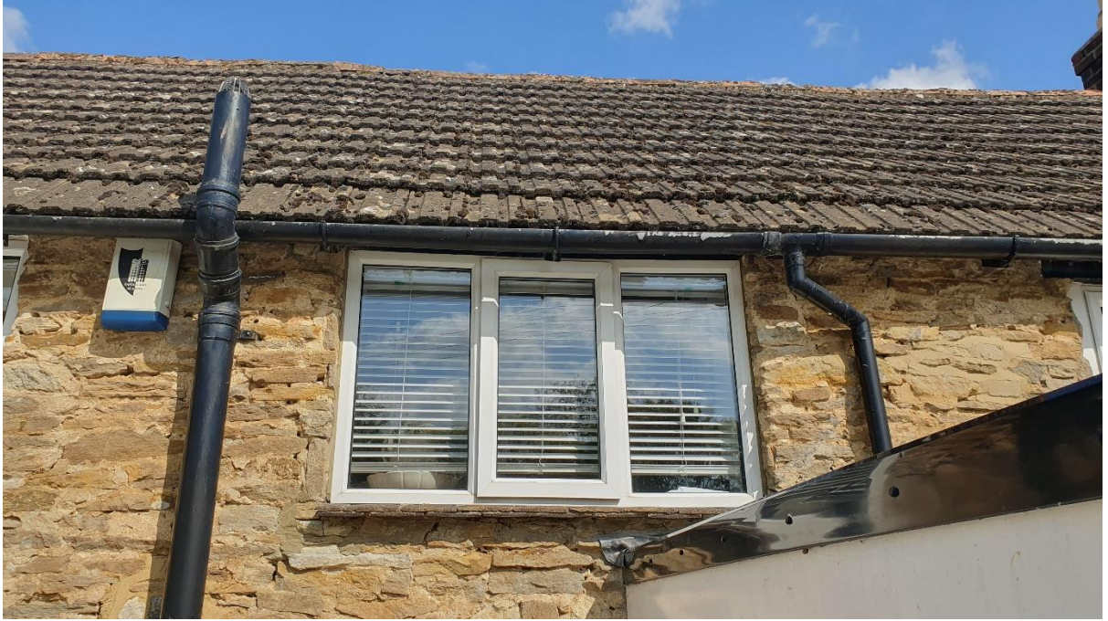
Image 11 – Existing window to No 1
