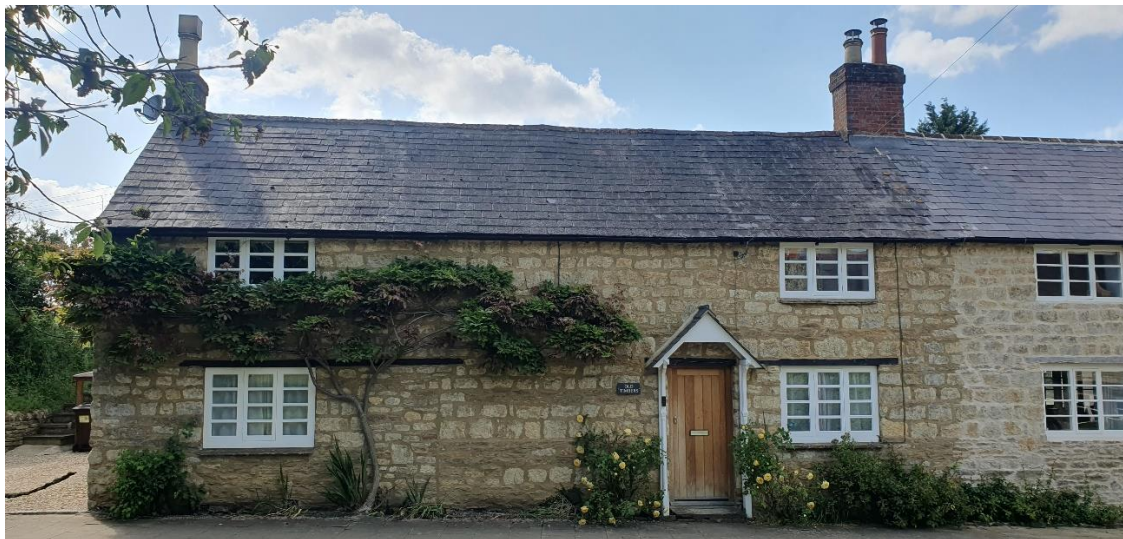
Image 2 – Photo showing the front elevation of No 1-2. Existing slate roof is to remain.
