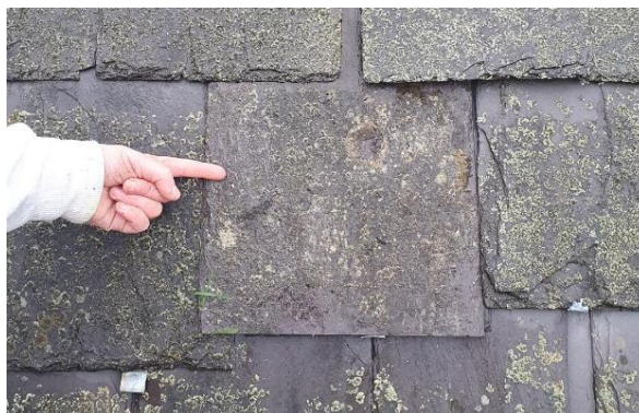
Image 4 - The sample purple slate was slotted into the roof of No 3-4 as part of its condition discharge requirement and provided a comparison of the replacement slates with the existing.
