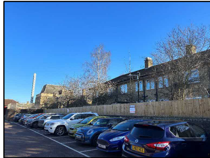
Photograph 1 View of Lambourne House from the adjacent car park
