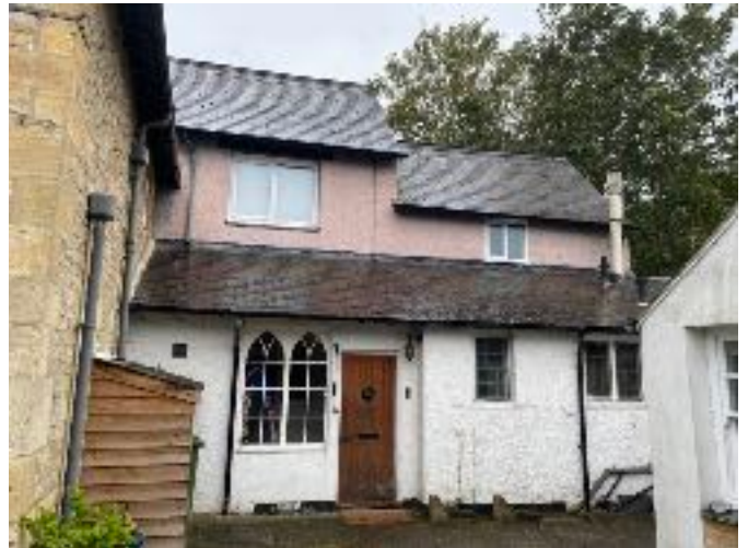
Existing - North Elevation (north entrance to main house).
