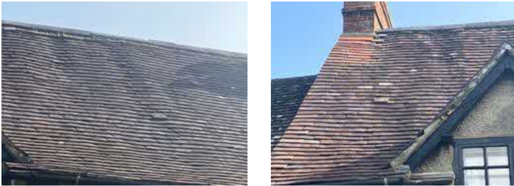
Figs. 7 & 8 Ridge and roof tiles to the front
