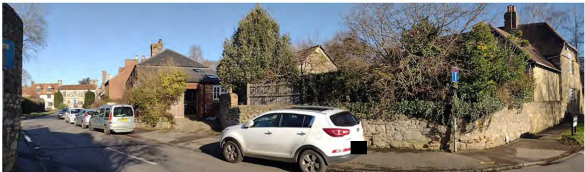
View from Junction of Mill Lane and Elsfeld Road. No's 1a and 1b Entrance path to right of brick garage abutting end of terrace, 1 Mill Lane.
