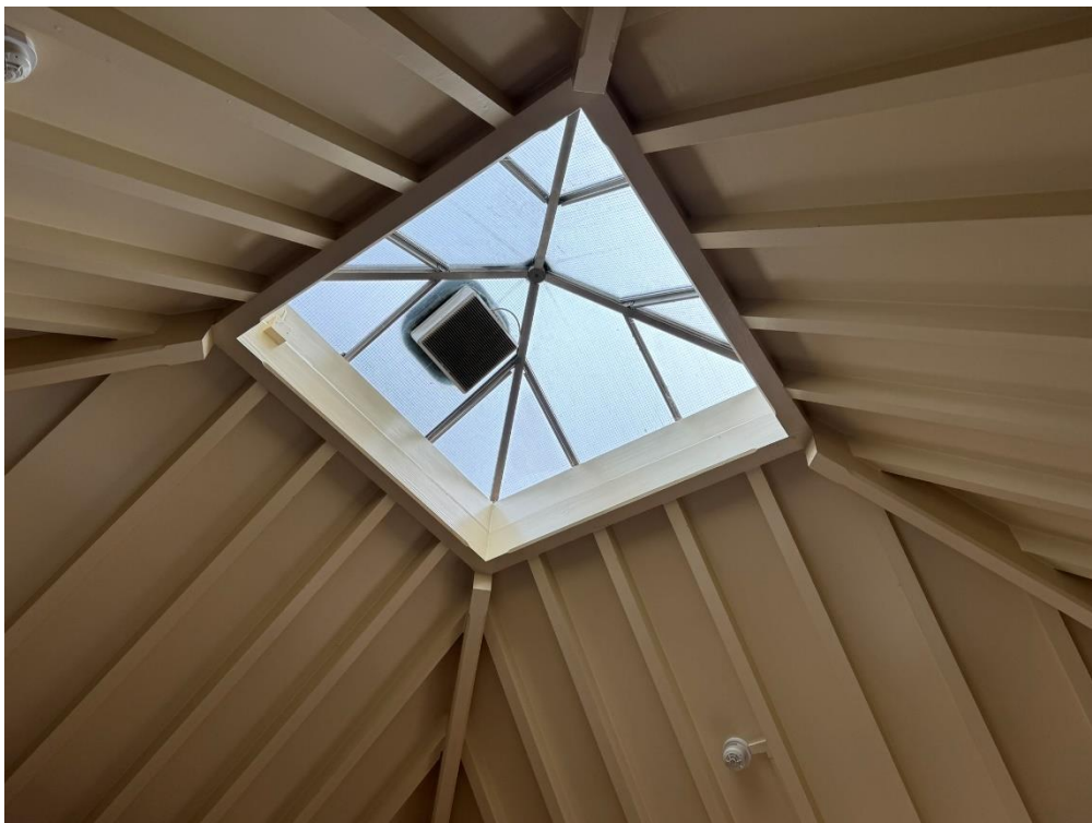
Fig.16 Existing roof Lantern to be replaced.
