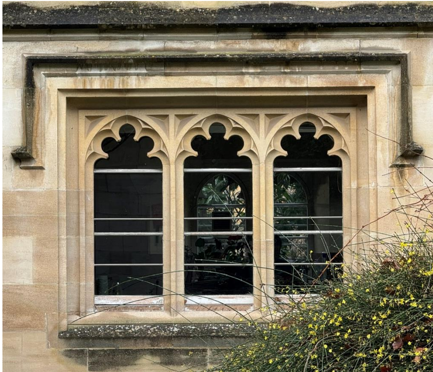
Fig.3 Existing 3-Light window to South East Elevation. Replacement window proposed to match existing.
