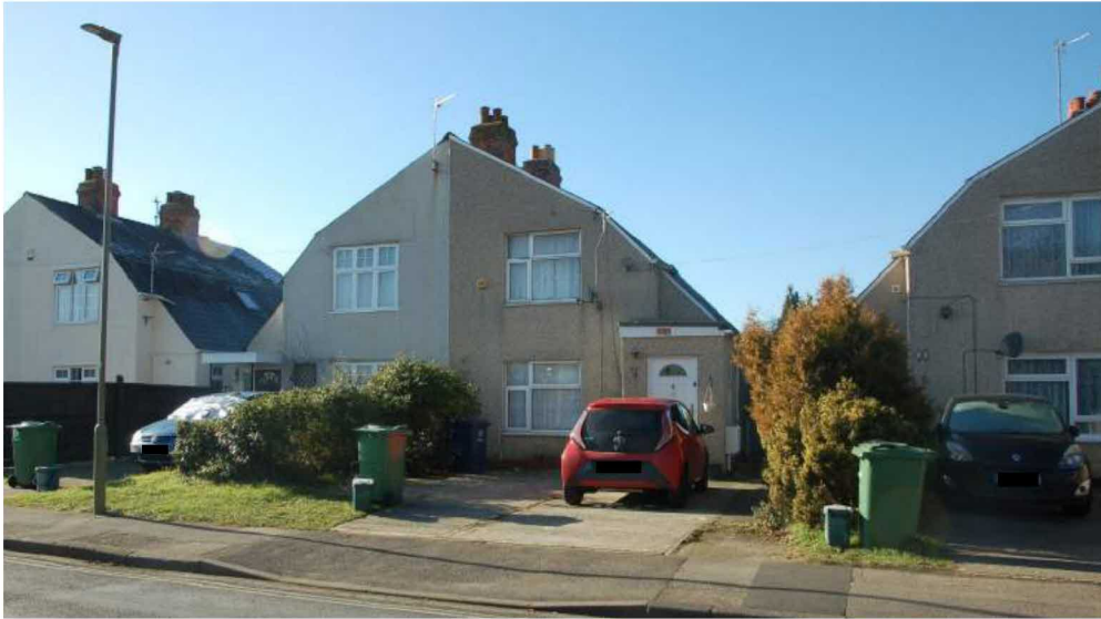
Porch extension at no. 25, Barton Road
