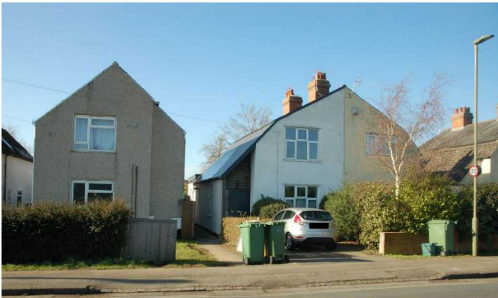
Porch extension at no. 7, Barton Road
