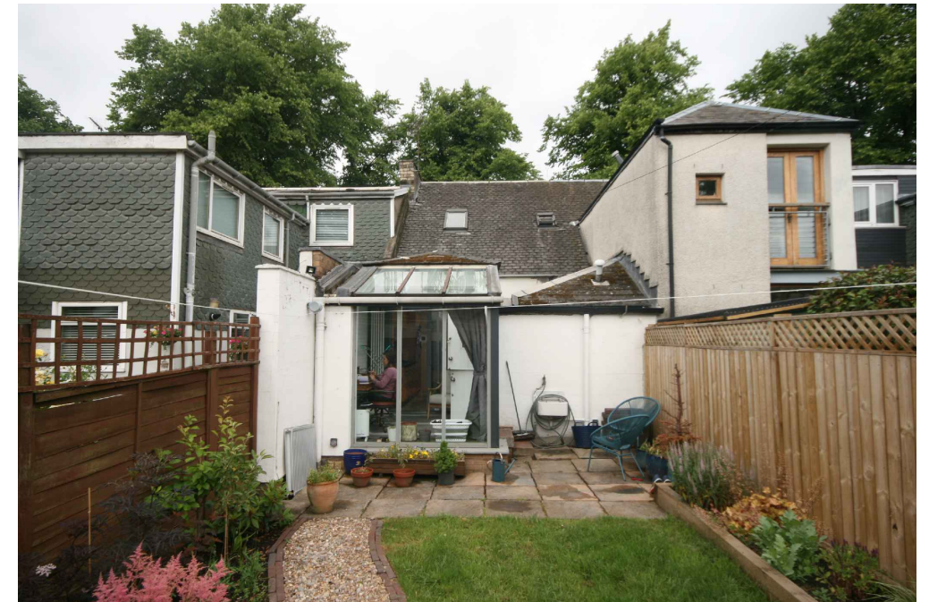
PHOTOGRAPH OF REAR AS EXISTING
