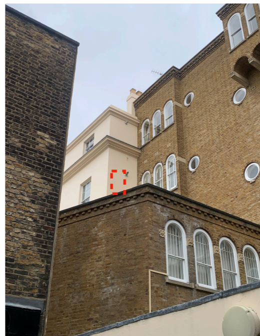
Rear facade for the new grille
