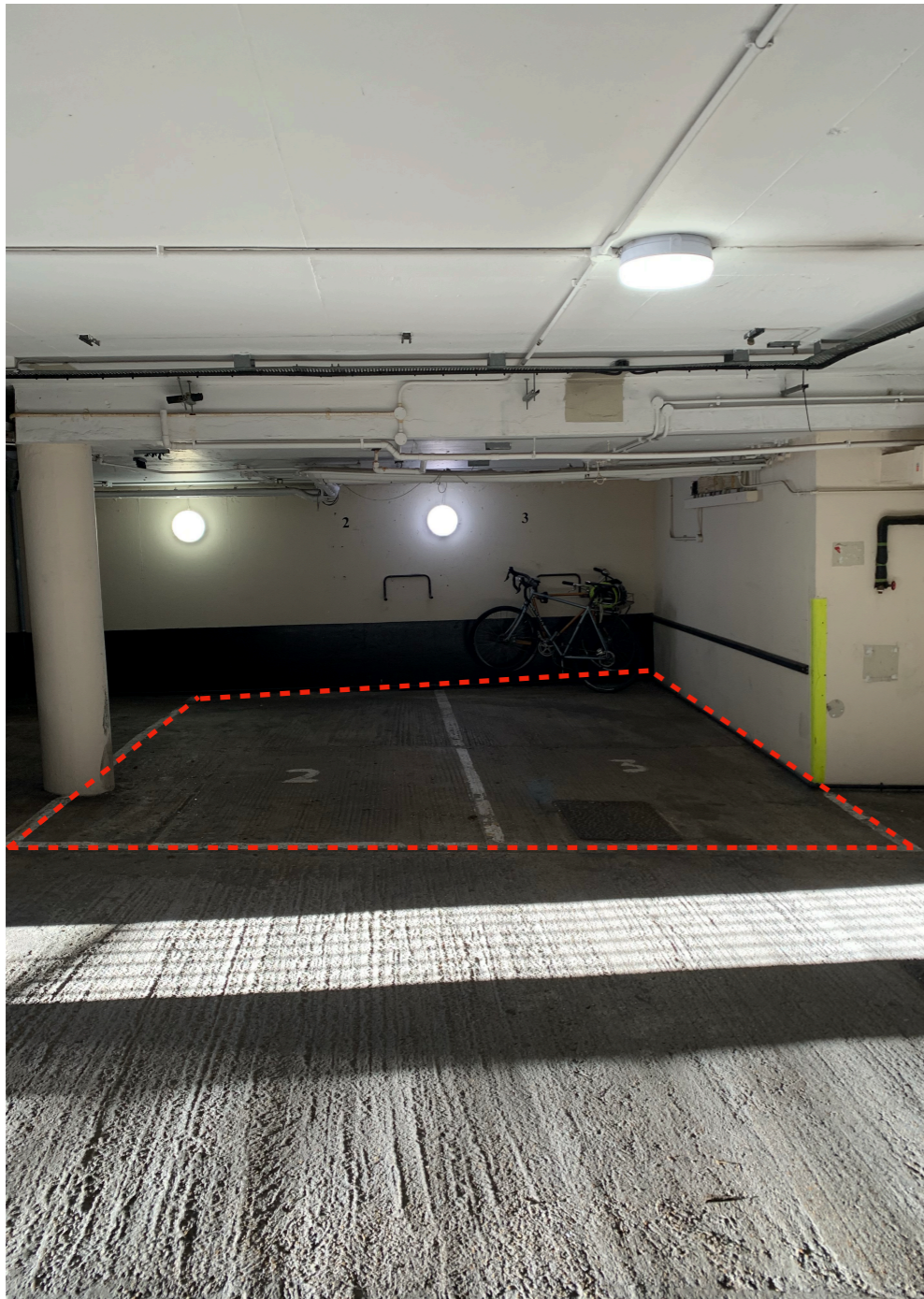
Existing basement carpark with Applicant's bays highlighted
