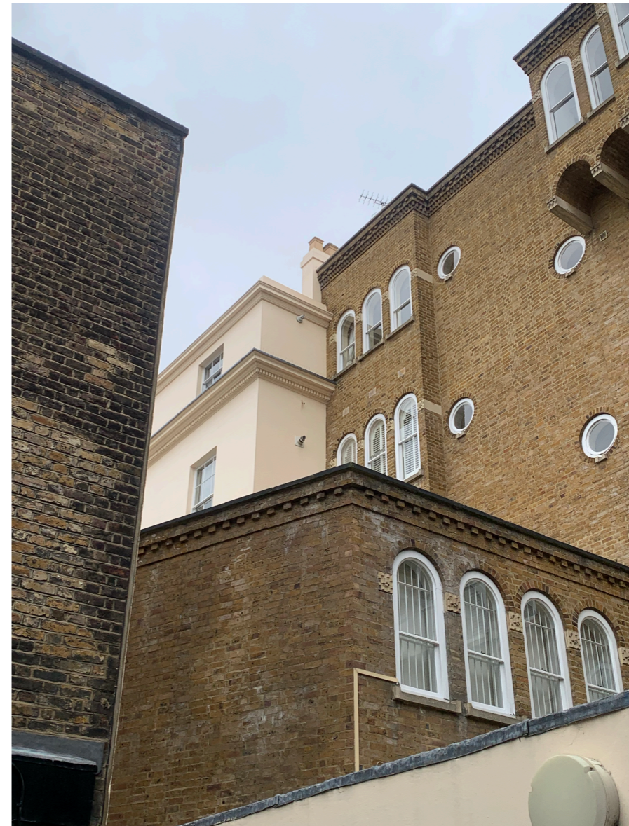
Figure 1 - View of existing rear facade
