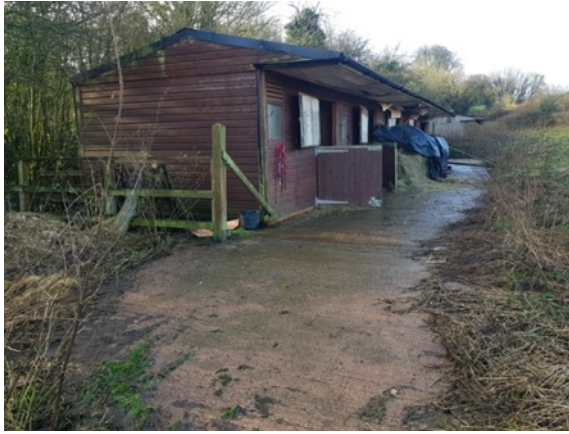
Photo 1: Stable block and concrete hardstanding located near the southern boundary of the site
