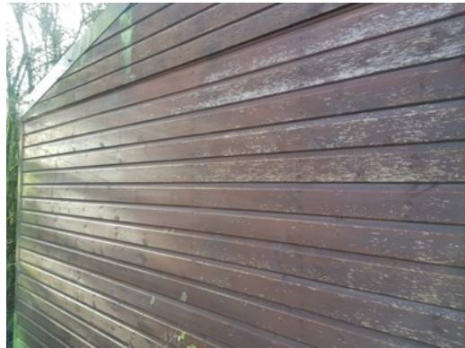
Photo 4: Timber clad elevations to stable block with no gaps or crevices
