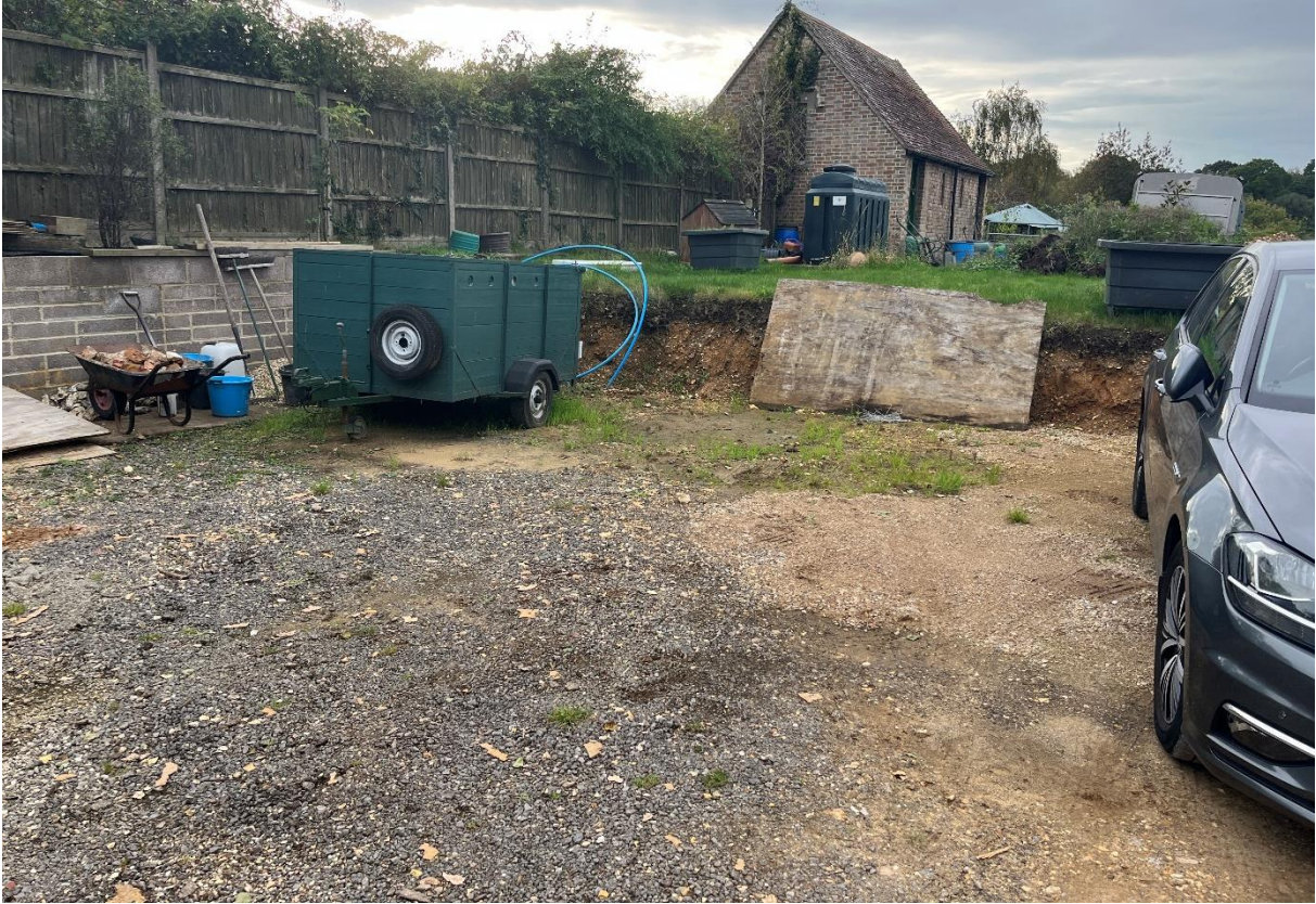
Photo 3: Excavation Works and Retaining Walls (Facing Rear Garden)
