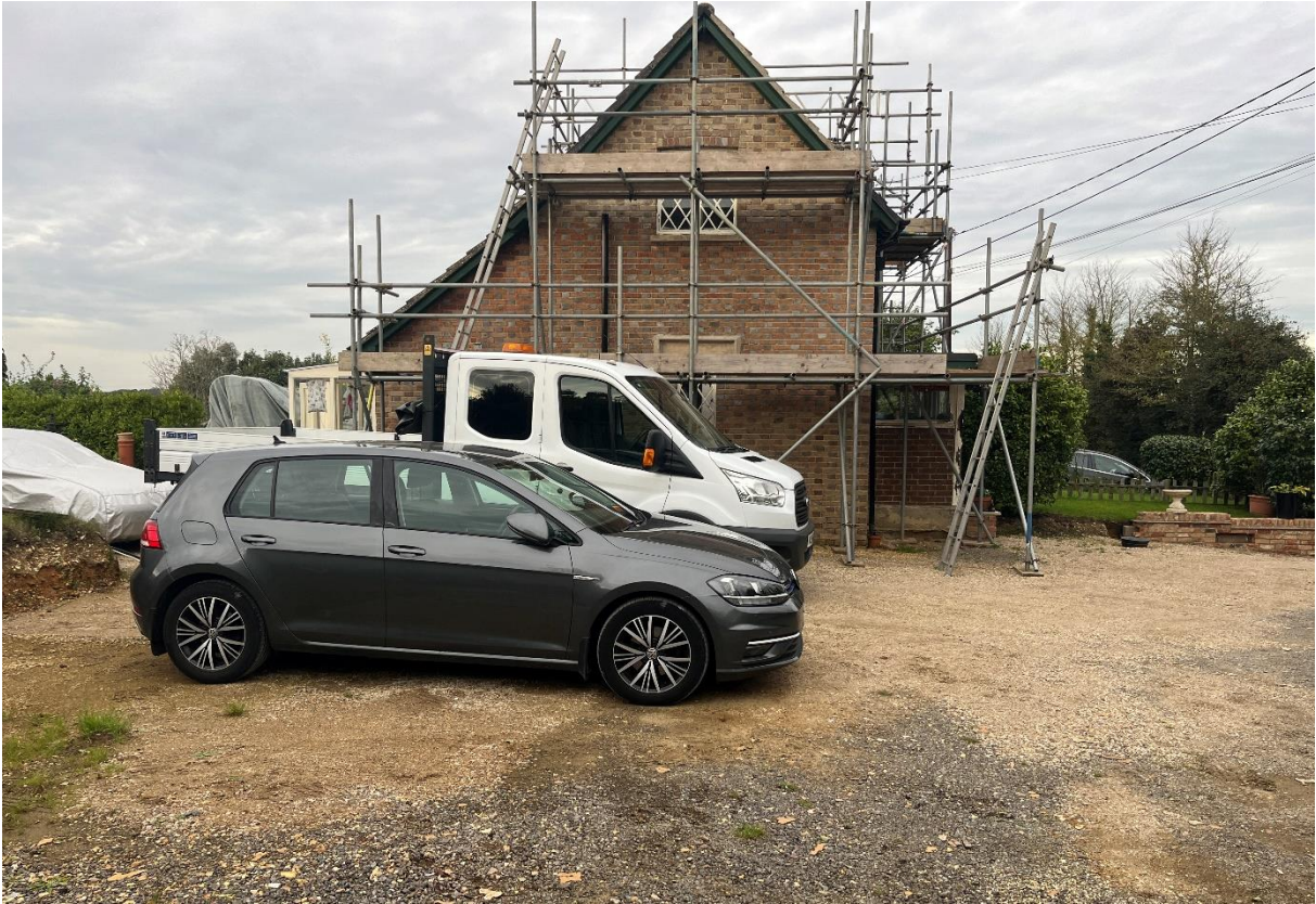
Photo 4: Parking Forecourt and Site Levels (Facing No 93 Ashington Lane)
