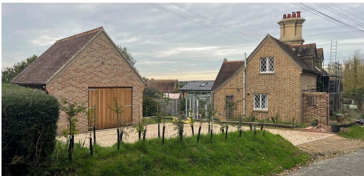
Fig 6: Photo of existing garage to the side of No 91 Ashington Lane.
