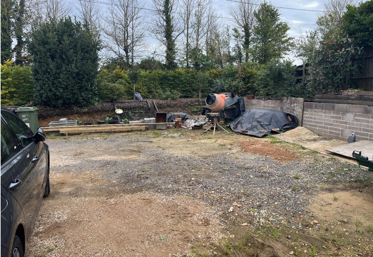
Photo 2: Excavation Works and Retaining Walls (Facing Ashington Lane)
