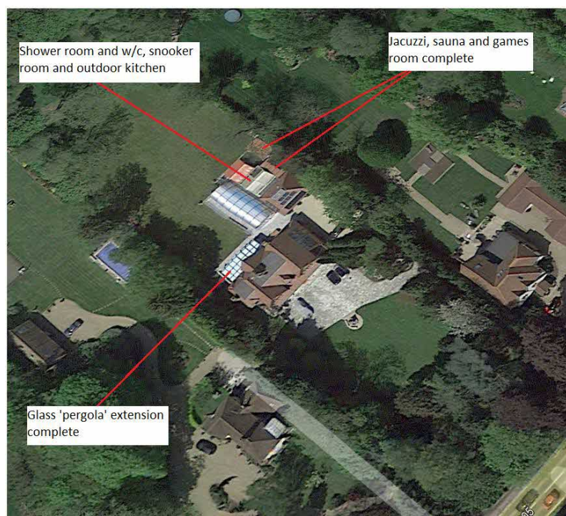
Google earth image July 2018; glass 'pergola' extension and outbuildings complete
