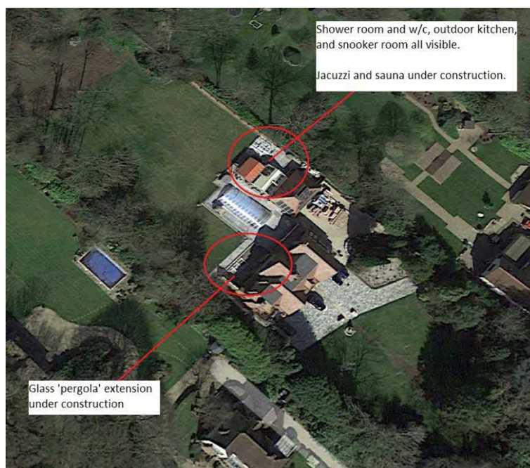
Google earth image March 2017; shower room and w/c, snooker room and outdoor kitchen existing. Jacuzzi and sauna under construction. Glass 'pergola' extension under construction
