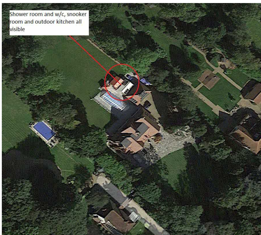
Google earth image March 2016; shower room and w/c, outdoor kitchen, and snooker room existing
