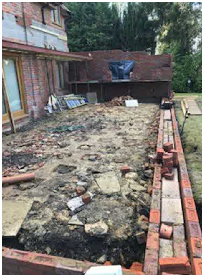
Photograph showing the pergola extension under construction (dated 7 February 2017)
