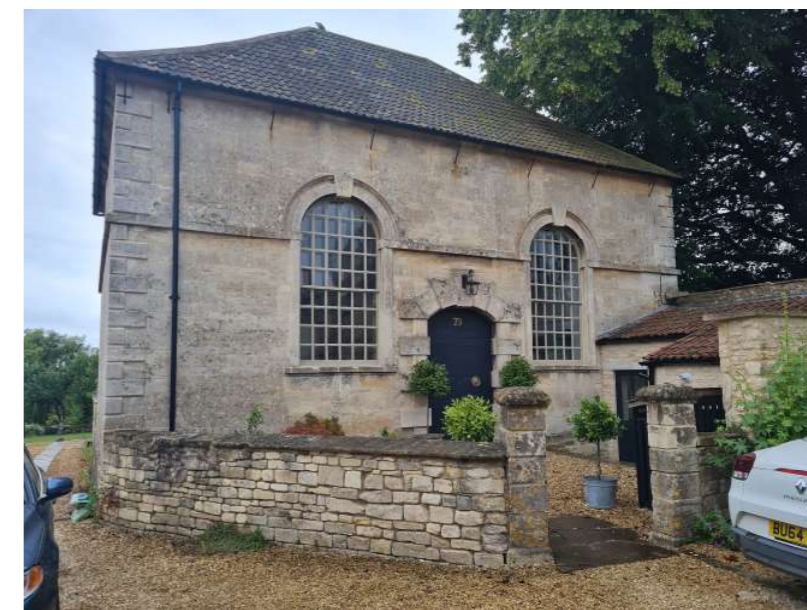
Fig 5. Photo of front elevation of host building showing area of proposed parking. Left hand gate pier and section of wall reduction shown in foreground.
