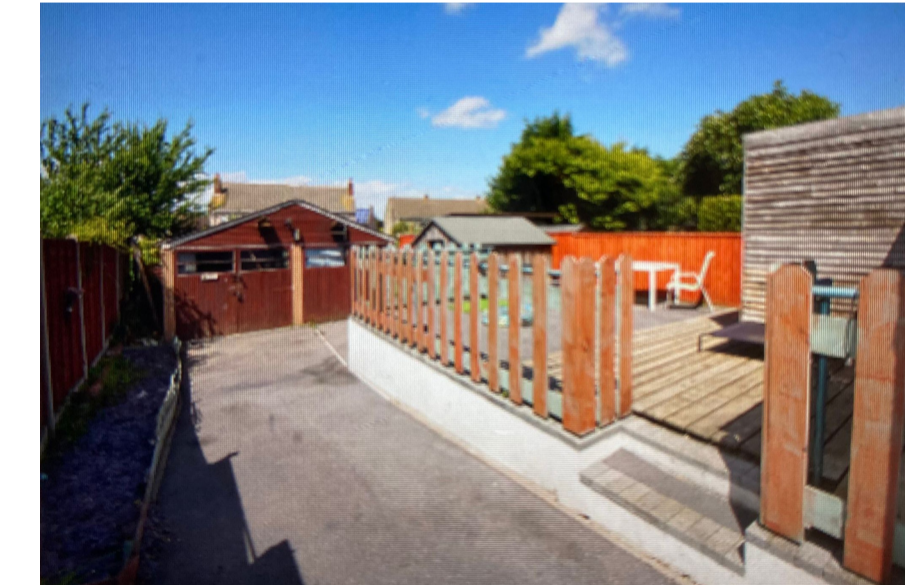
PREVIOUS LARGE SHED STRUCTURE TO REAR GARDEN - THIS HAS SINCE BEEN REMOVED
