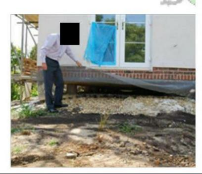
The completed deck with pile overlays made of flexible material prevents concrete from the slab pour leaching onto the ground surface. Similarly the aluminum strips between the sheets of ply prevent concrete reaching the ground surface.
