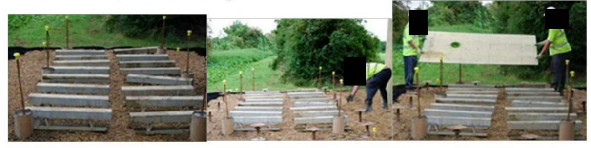
Perimeter jacks are laid around the edge of the footprint to allow fine level adjustments to be made.
