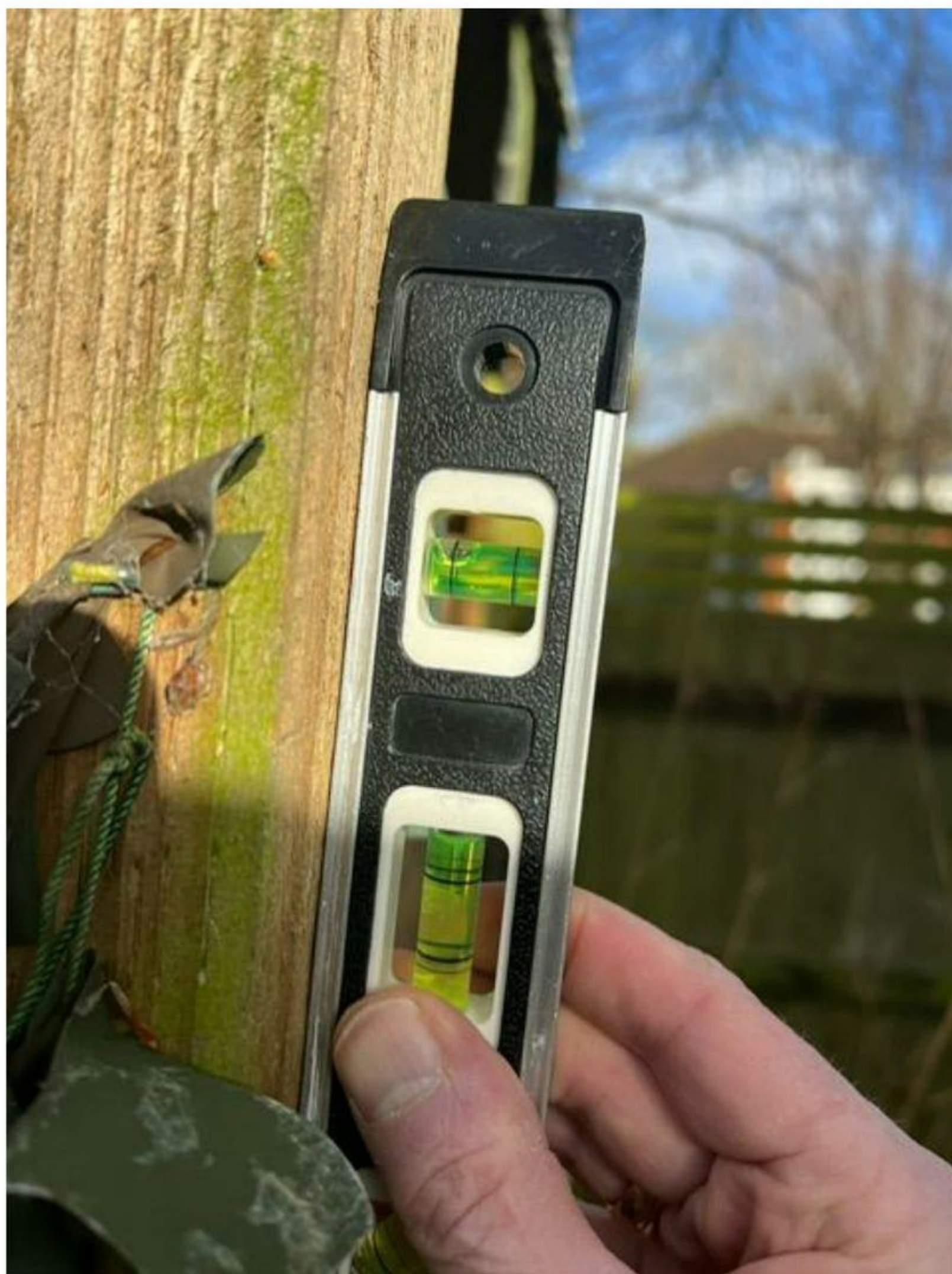
Photo 6 – Fort legs now leaning off centre.
