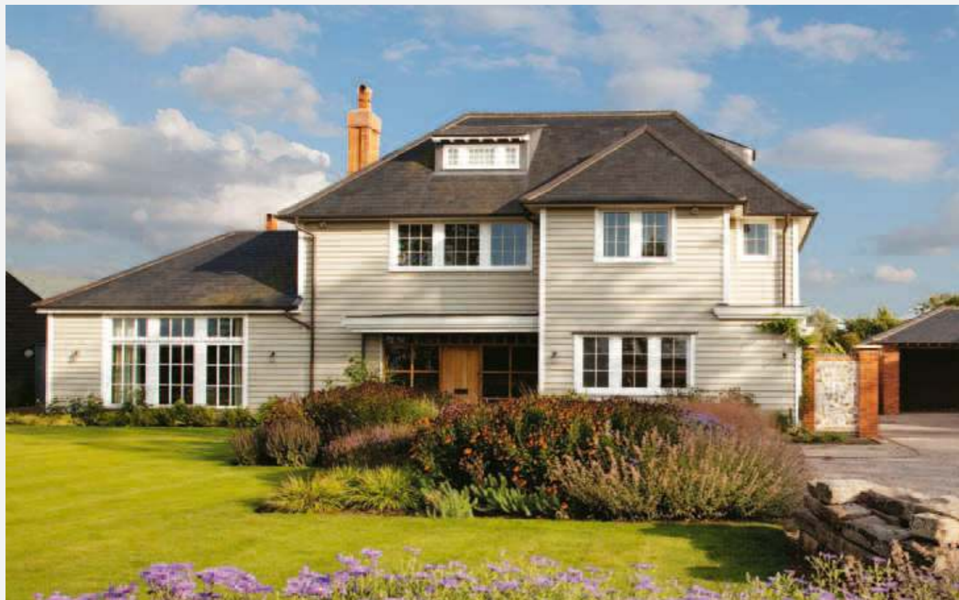
Newly built family home includes Casement Windows in Westbury White
