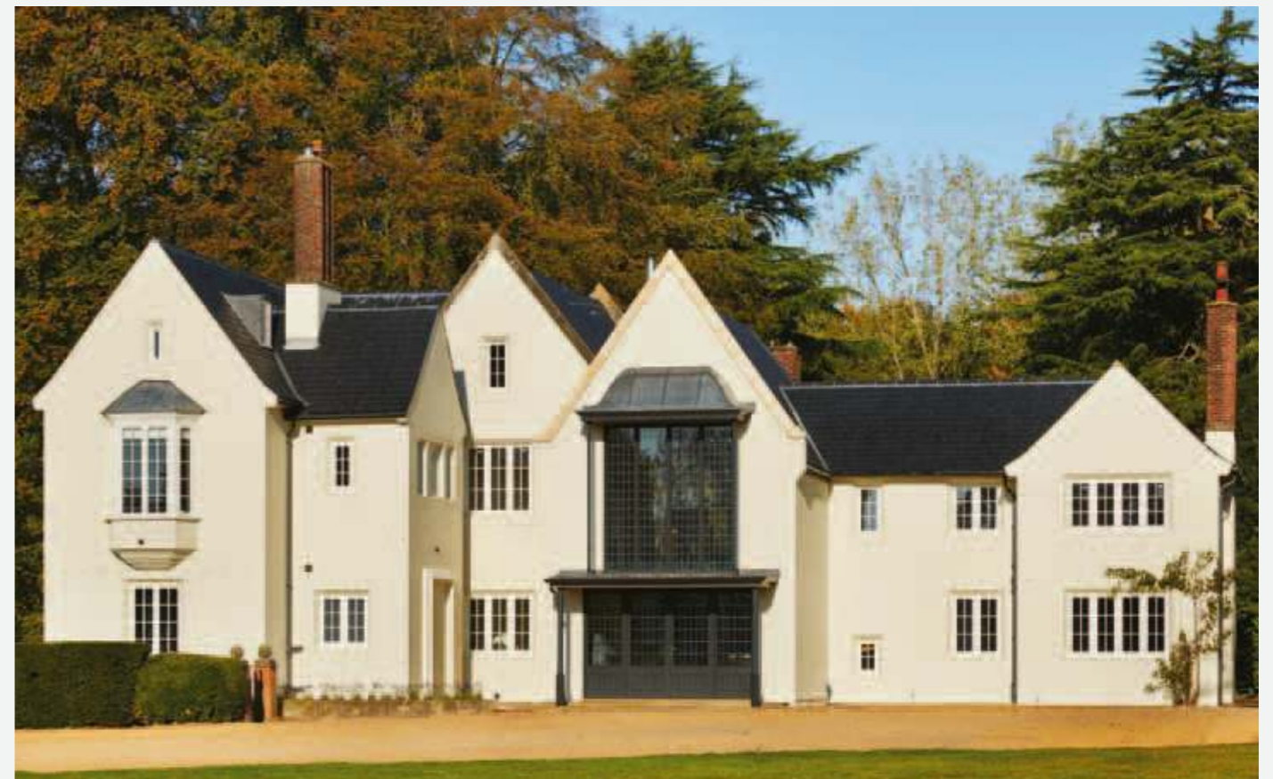
Refurbishment project with Casement Windows complemented by Engineered Oak Screen with antique lead glass design, in bold Westbury Black
