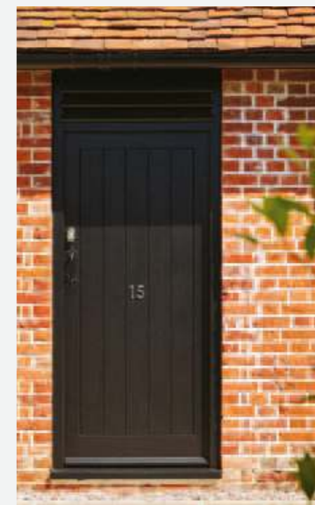
Boarded Entrance Door COLOUR: Westbury Black
