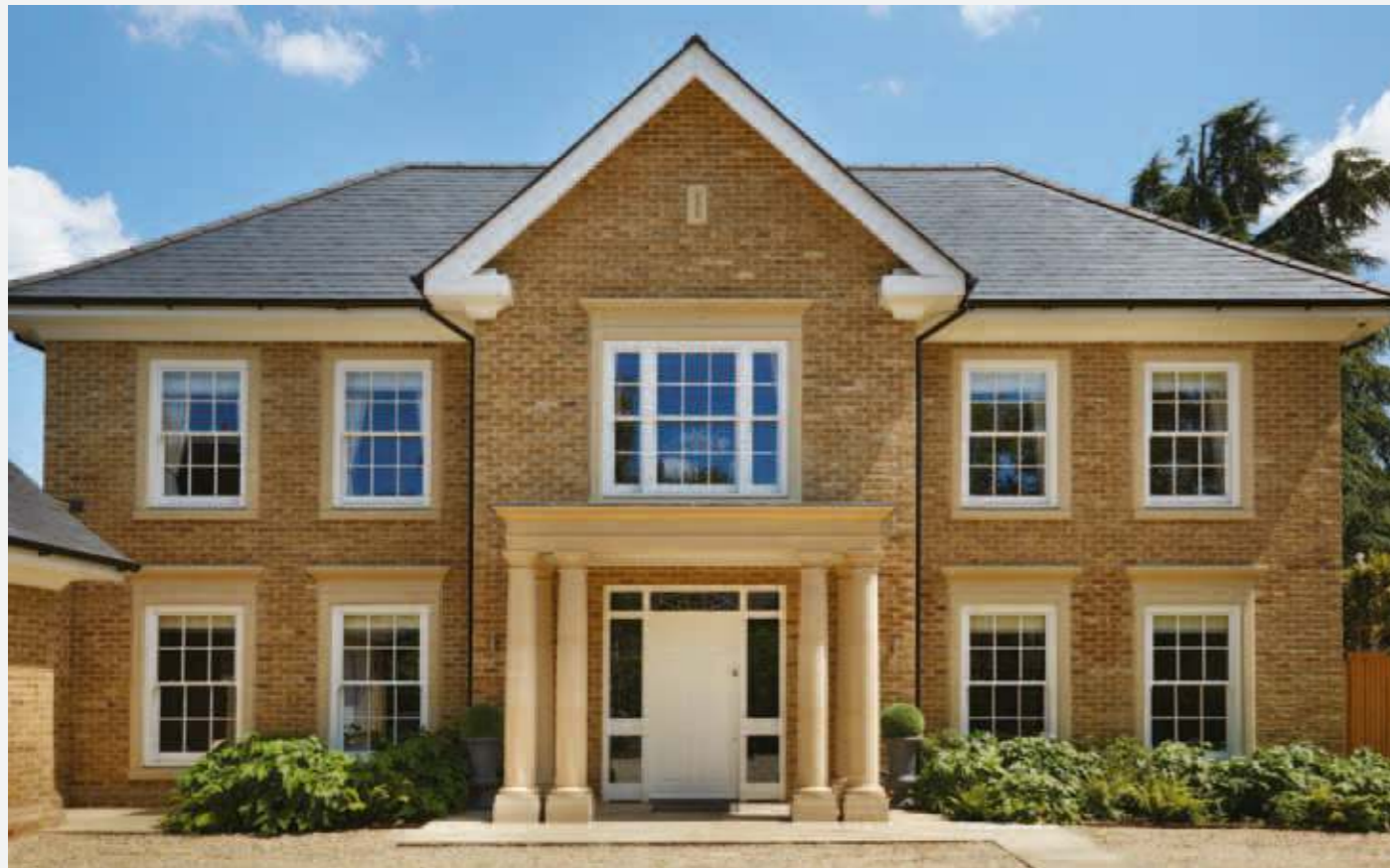
Spring Balanced Sash Windows and 6 Panel Entrance Door
