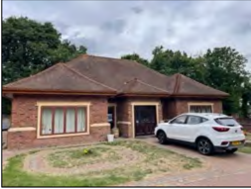
Photograph 1: The eastern elevation of building B1.
