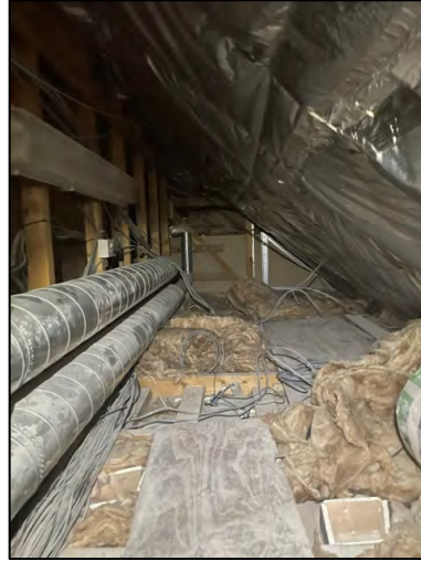
Photograph 2: The western roof void of building B1.
