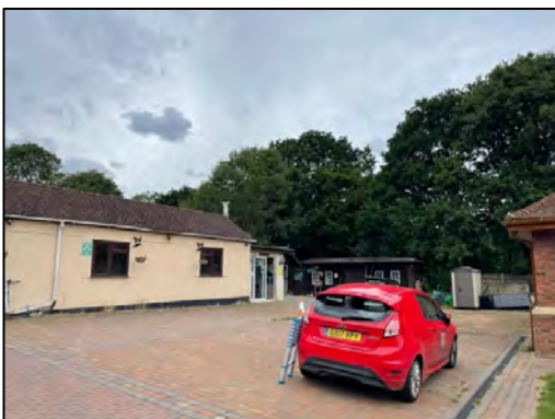
Photograph 15: The northern elevation of building B4. Building B5 can be seen in the background.
