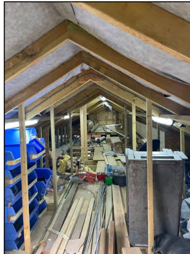
Photograph 4: The main roof space of building B2.
