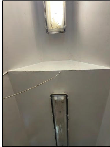
Photograph 6: The inaccessible roof void of building B9.
