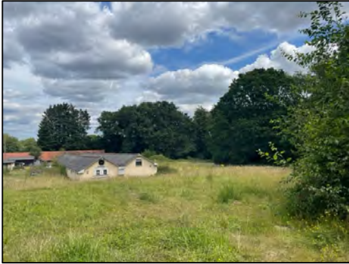
Photograph 5: The north-eastern aspect of the Site. Building B9 can be seen in the centre of the photograph. Photograph taken from the south-eastern aspect.
