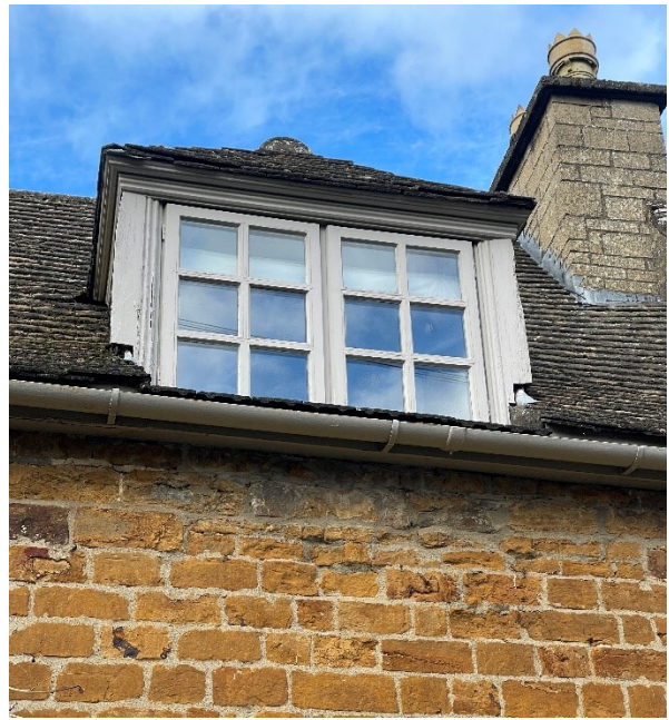
First Floor Window example
