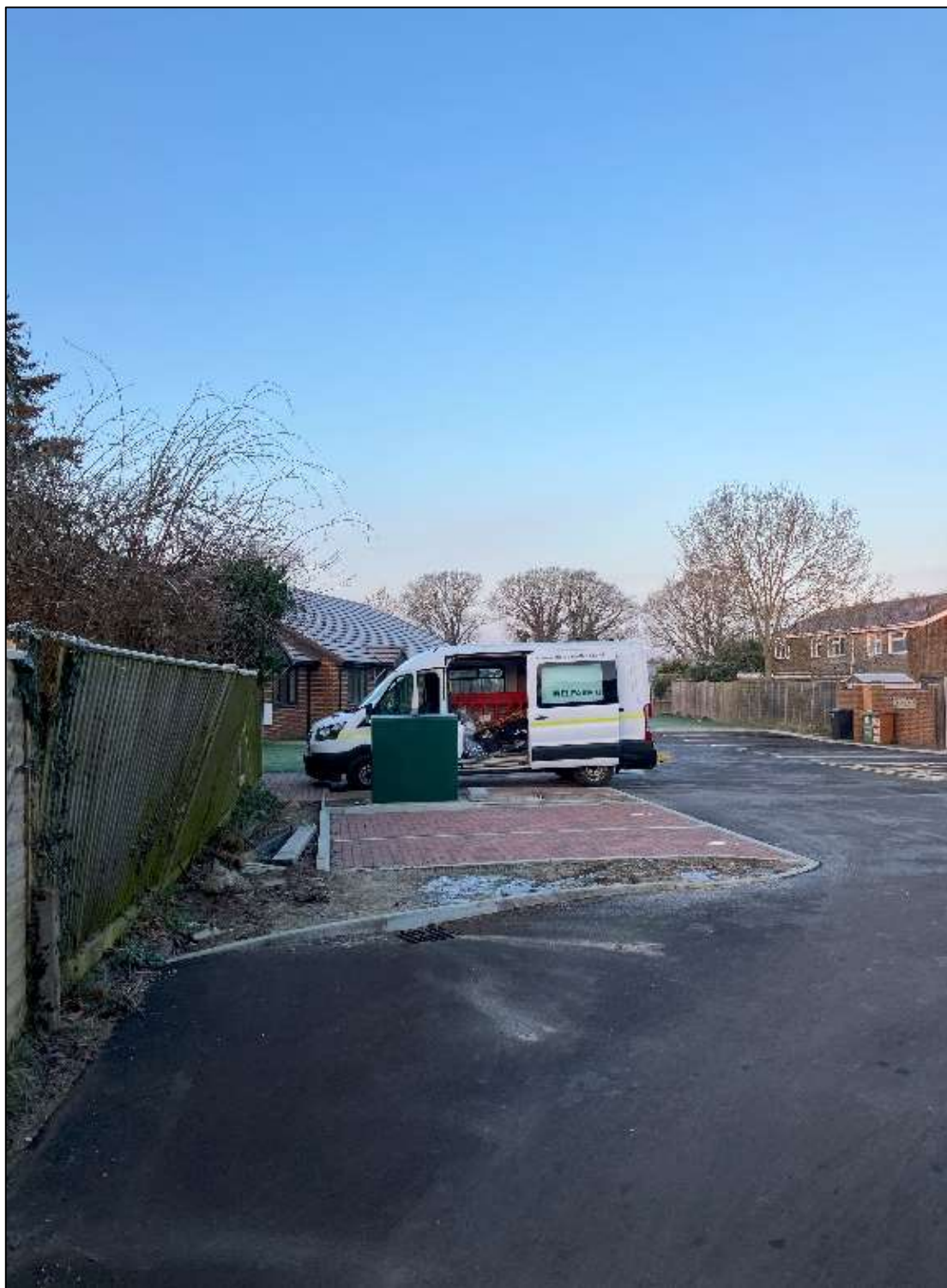
Photo 1 – Site entrance facing west
