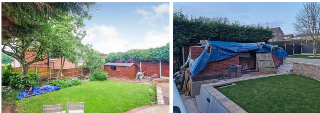
Figure 4 Original shed in situ and part-built outbuilding.
