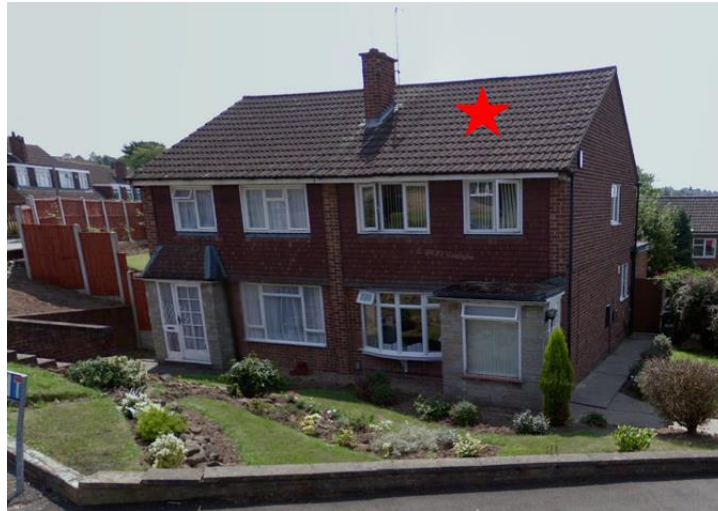
Figure 1 View of the front of the property from Connolly Close.
