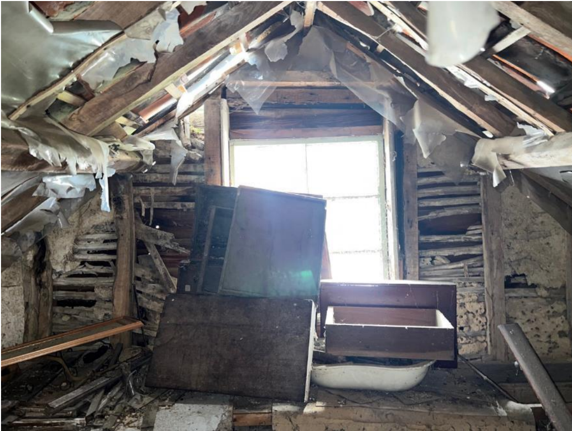
Photo 36. Shows wattle and daub on southern end of barn. Above B1.
