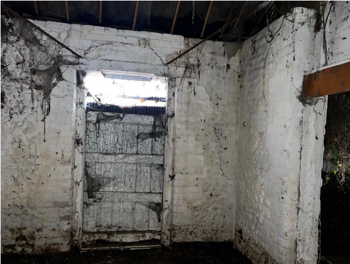
Photo 28. Internal view of The Barn, section B6.
