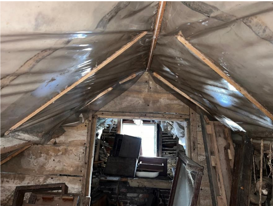
Photo 41. Shows loft space and plastic sheeting.
