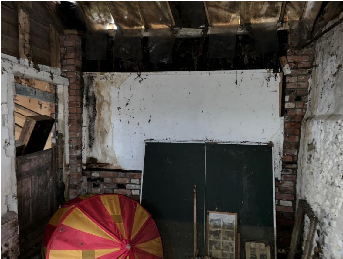
Photo 30. Internal view of The Barn, section B6. Looking west.
