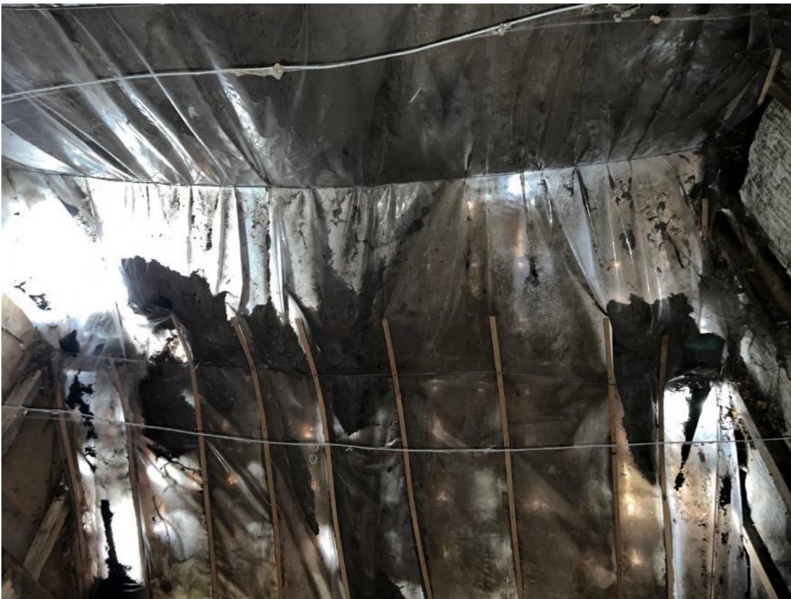
Photo 29. Internal view of The Barn, section B6
