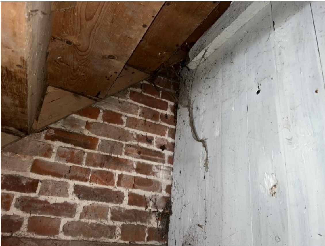
Photo 20. Internal view of the barn, section B3.
