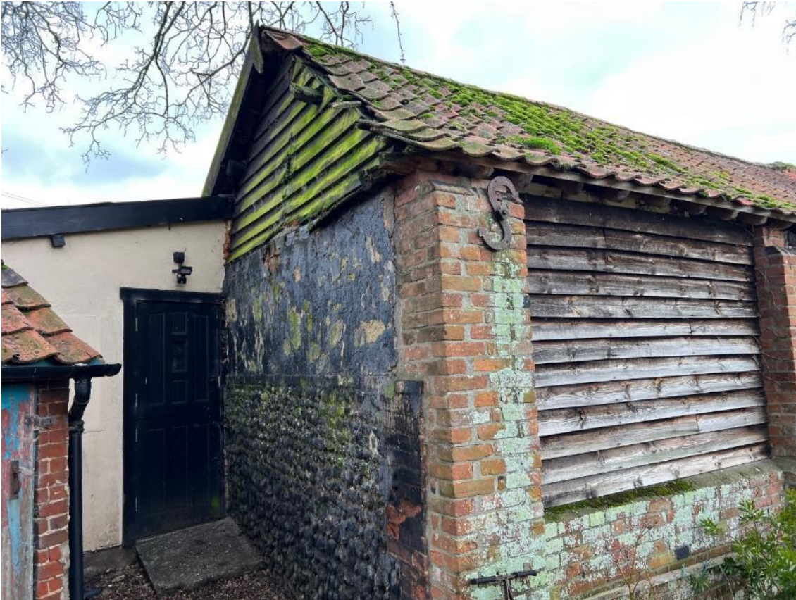
Photo 32. Shows barn, section B6 and adjoining store. Looking east.
