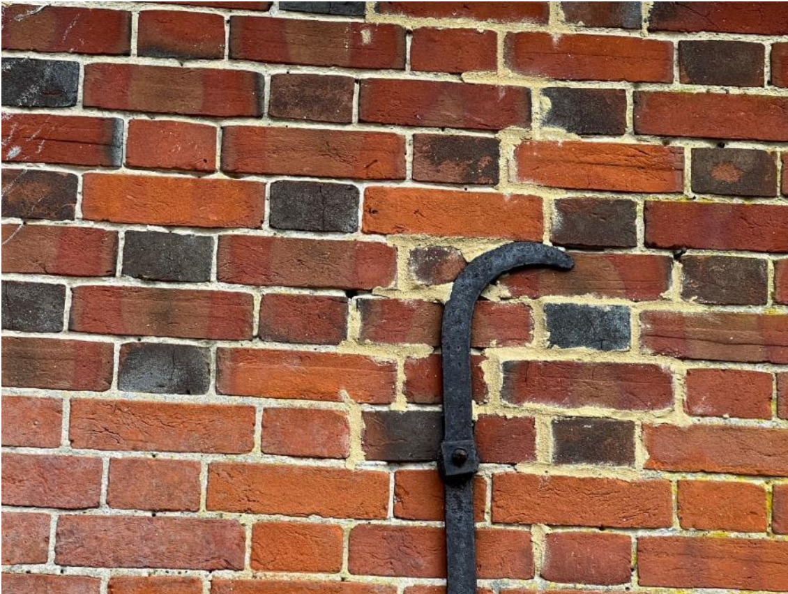
Photo 21. Shows metal tie support on rear of barn (west aspect).
