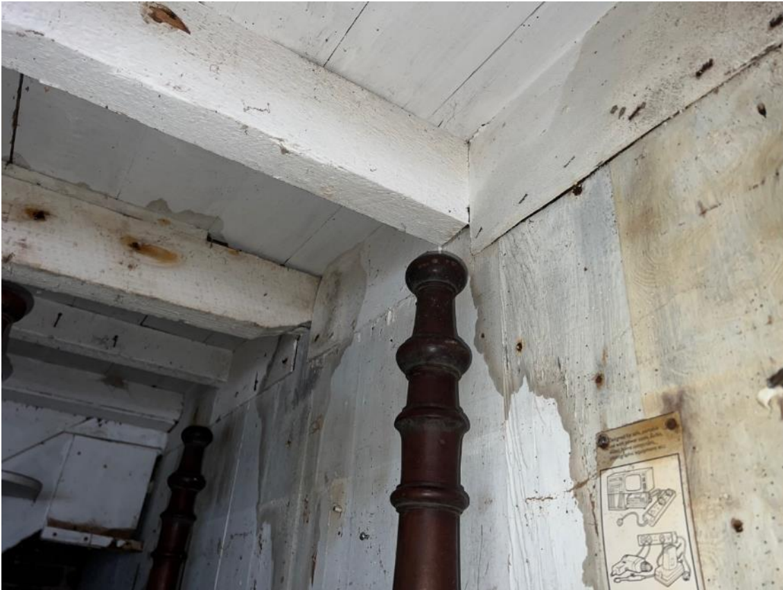
Photo 19. Internal view of the barn, section B3.
