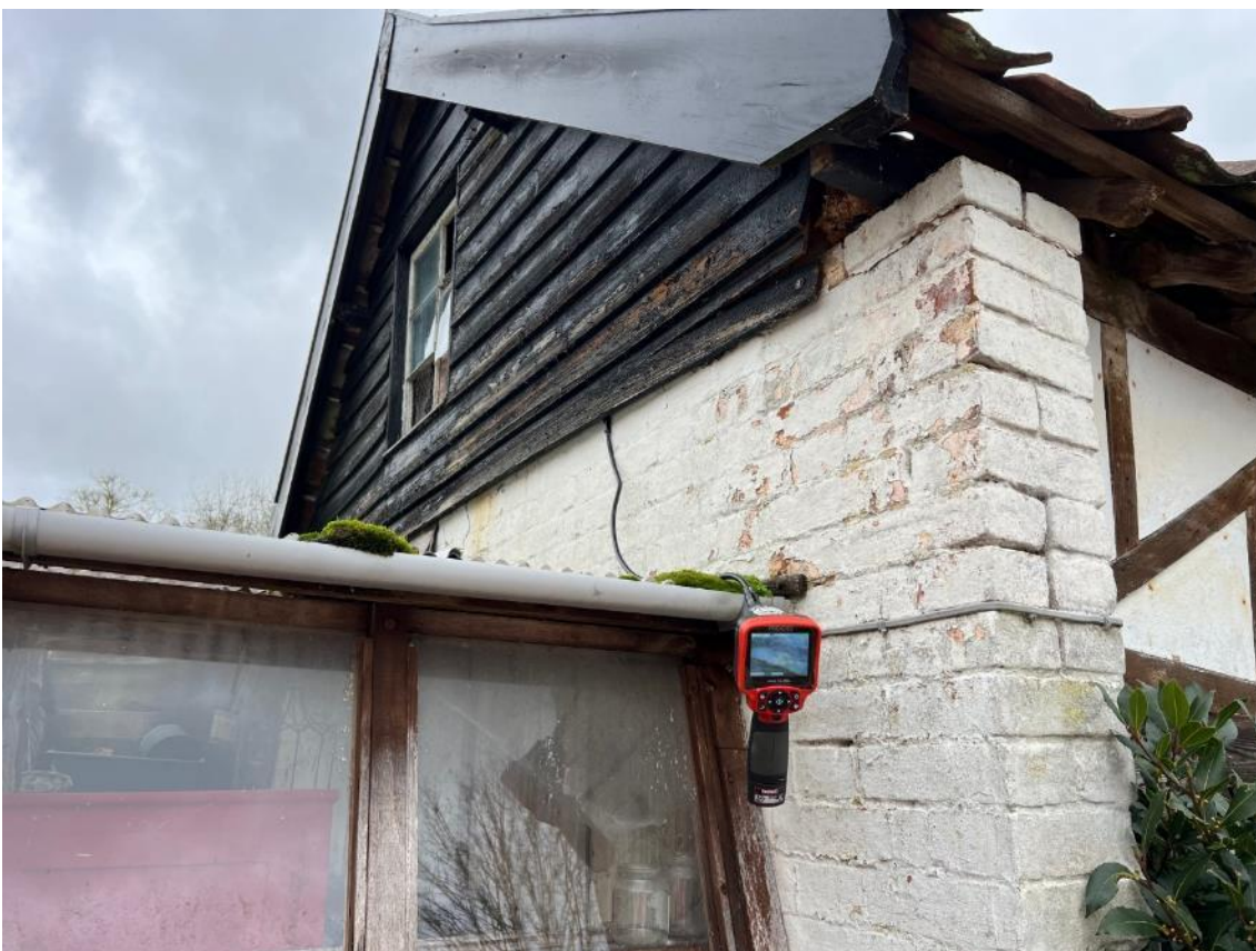
Photo 16. Shows endoscope being used to explored under the external timber cladding on the south gable wall of the barn, B1.
