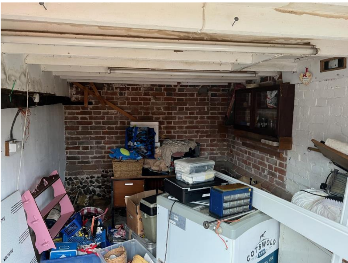
Photo 21. Internal view of The Barn, section B4.
