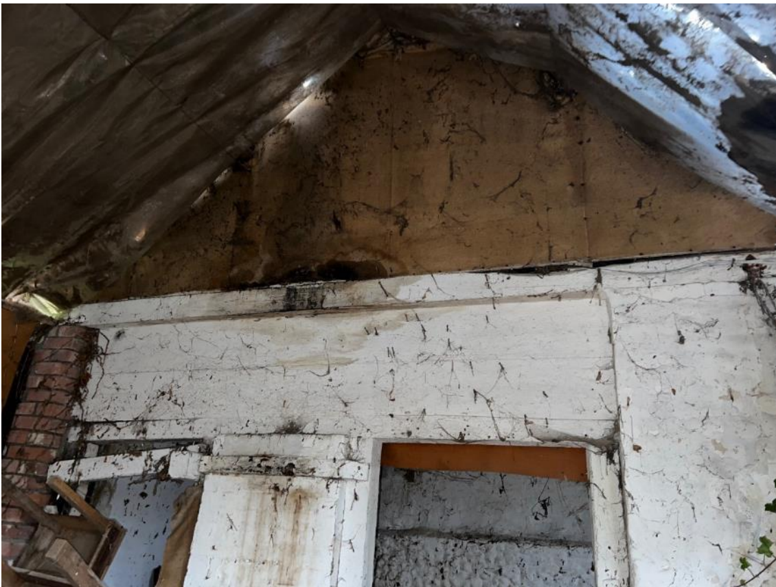
Photo 27. Internal view of The Barn, section B6.
