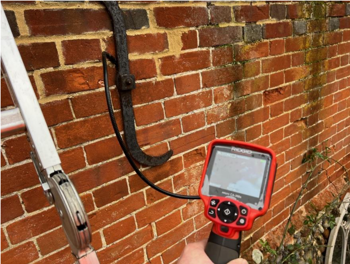
Photo 44. Inspecting small gap behind metal tie support.
