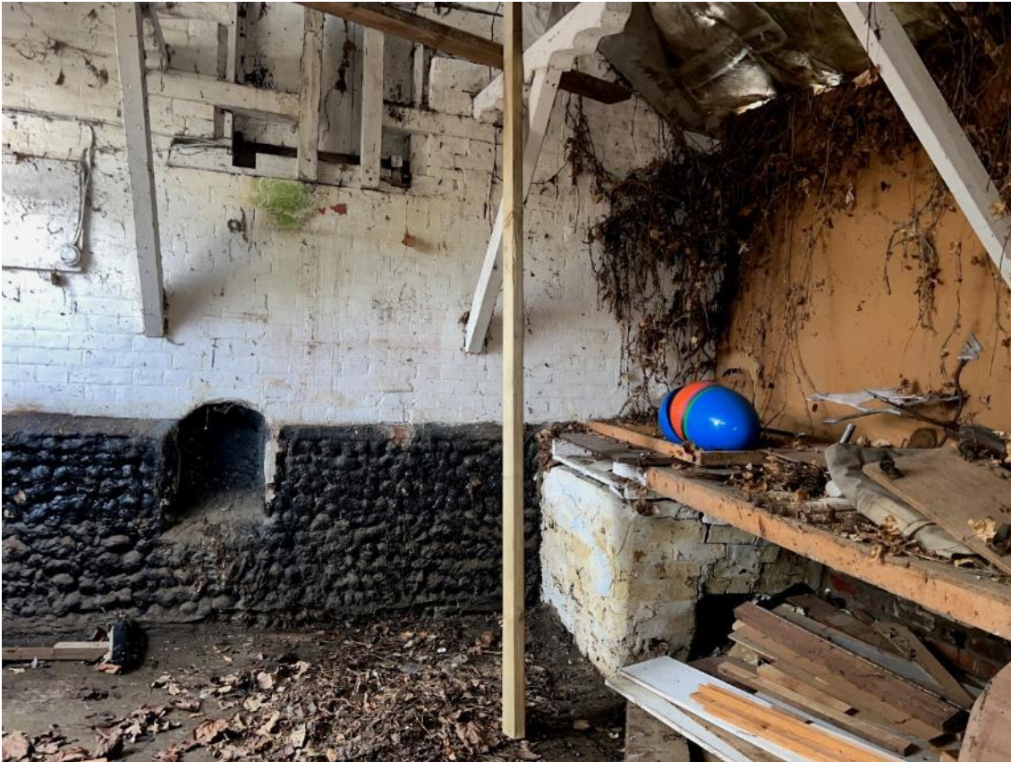
Photo 26. Internal view of the barn, section B5.
