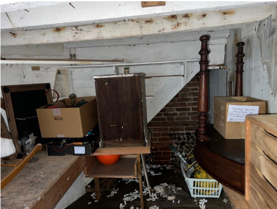
Photo 18. Internal view of the barn, section B3.
