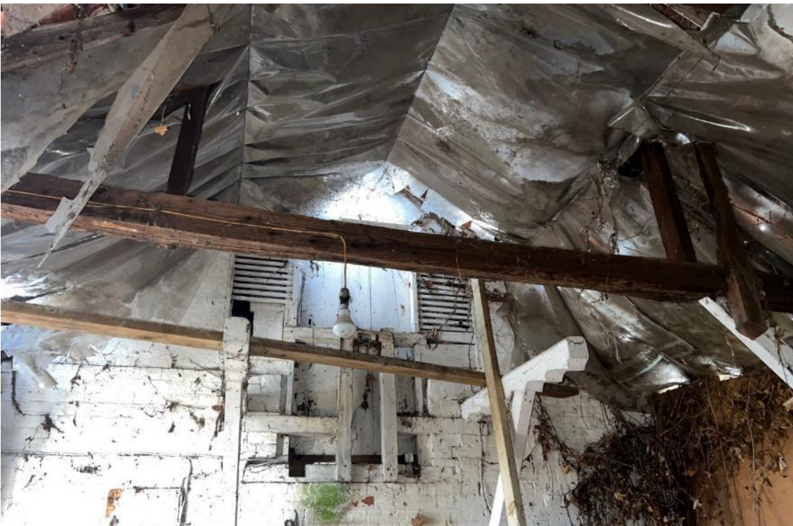
Photo 25. Internal view of the barn, section B5.
