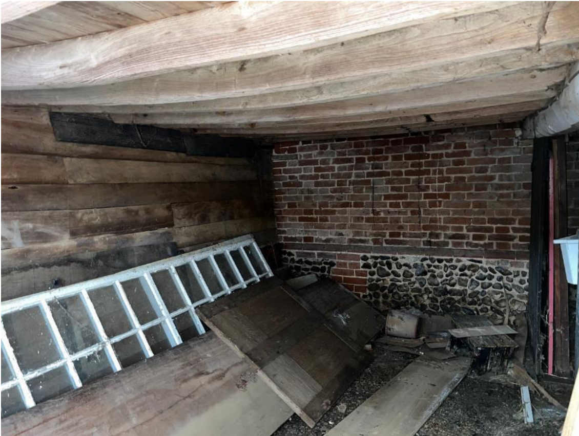
Photo 17. Internal view of The Barn, section B2.
