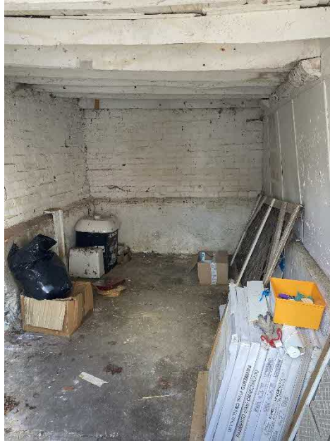
Fig 12 – Internal view of floor joists supported by dividing wall.
