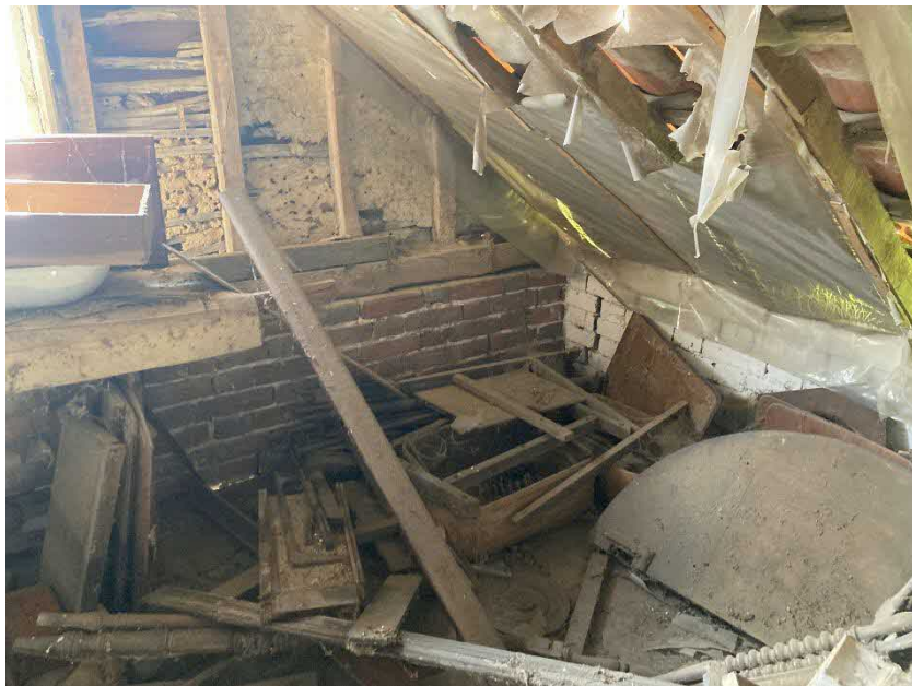
Fig 9 – Internal view of first floor gable wall & rear elevation.
