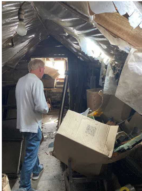
Fig 6 – Internal view of roof structure in two storey section.
