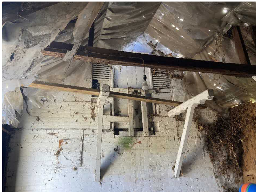
Fig 7 – Internal view of roof structure in single storey section.
