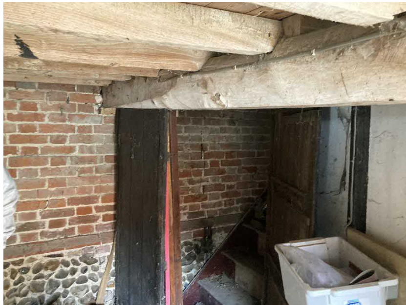
Fig 13 – Internal view of first floor downstand beams.
