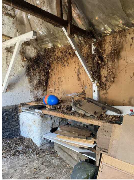
Fig 10 – Internal view of single storey rear studwork.
