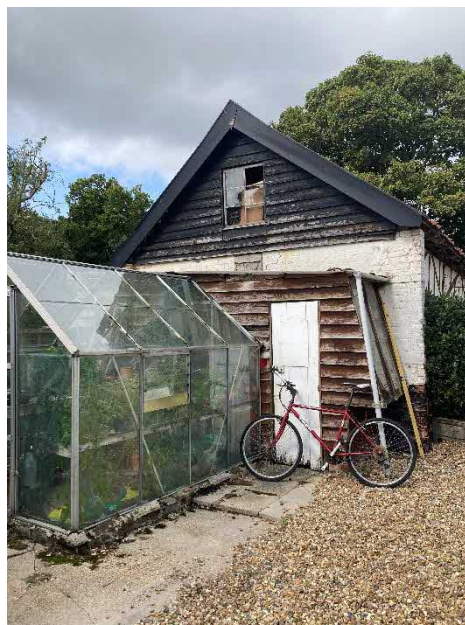
Fig 2 – South-East Elevation – Gable end of existing outbuilding, viewed from driveway.
