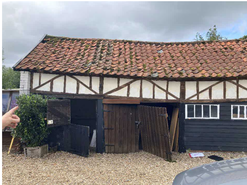
Fig 11 – External view of studwork over doors in front elevation.
