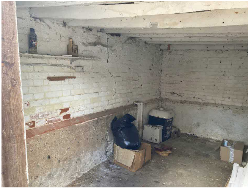
Fig 8 – Internal view of ground floor gable wall & rear elevation
