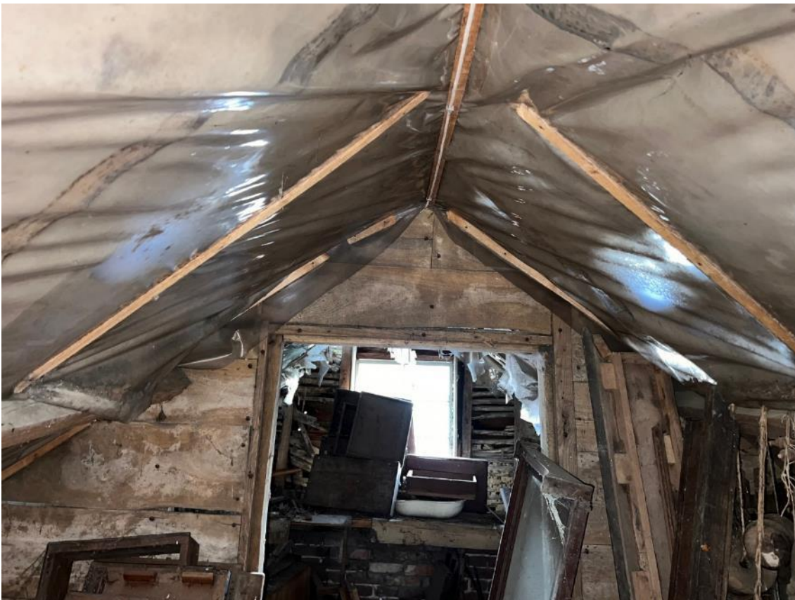
Photo 41. Shows loft space and plastic sheeting.
