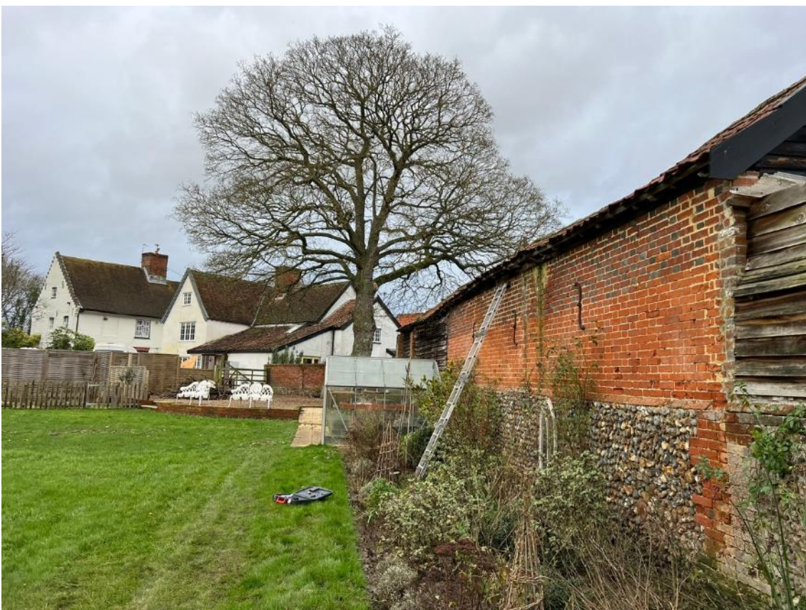
Photo 10. Shows west aspect of the barn.
