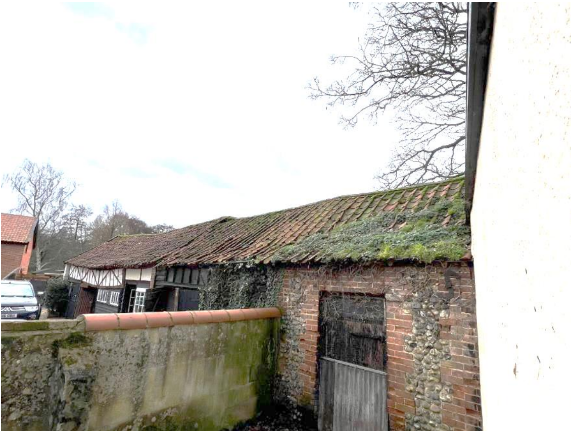
Photo 3. Barn. East aspect. Shows brick wall adjoining barn.
