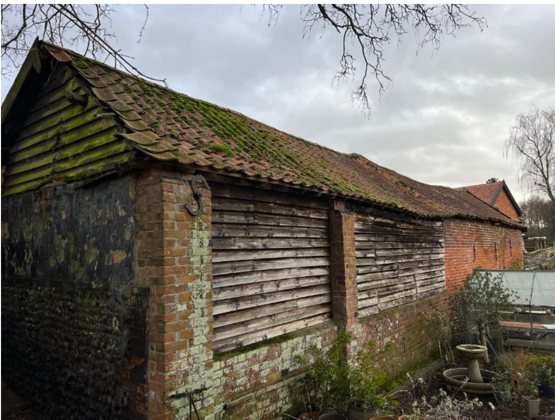
Photo 33. View of the barn, b6. West aspect.
