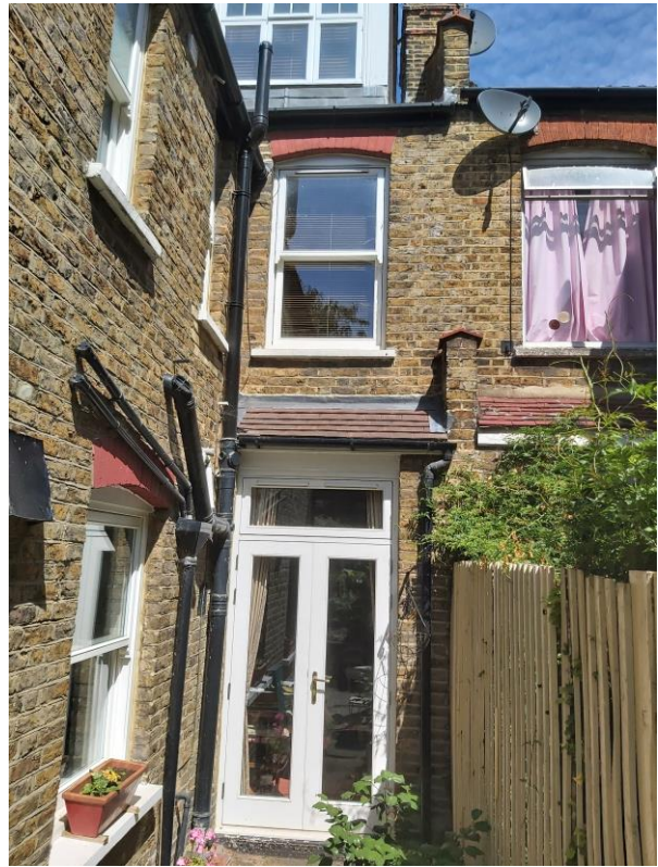
Fig.4 View of side passage and existing 2.1m height fence with no. 38
