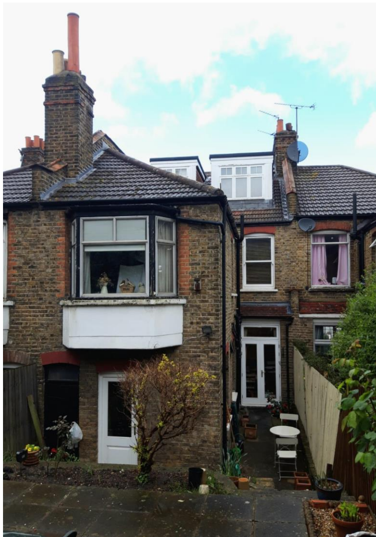
Fig.1 Photo showing rear elevation of existing property
