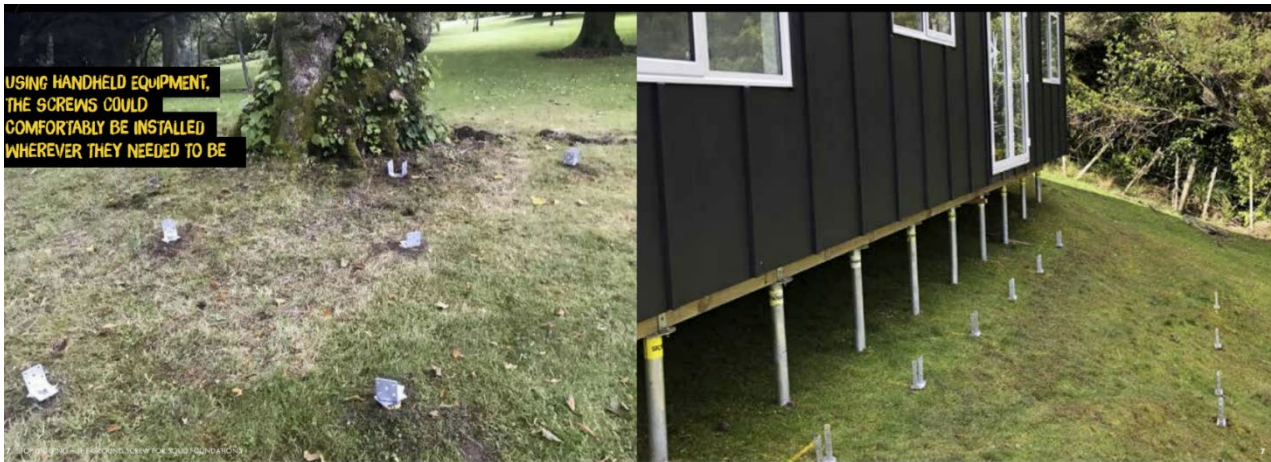
Figure 3: Stop Digging ground screws
