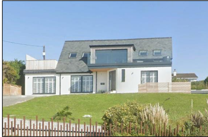
Neighbouring dwelling to the north-west of the site
