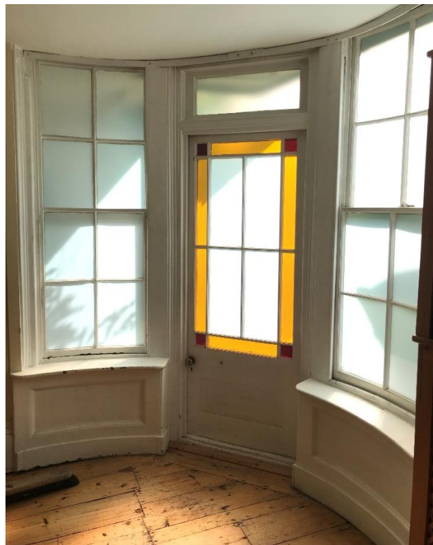
Figure 14: Internal elevation of the curved quadrant bay window – the door and right-hand sash window are modern replacements within what appears to be a 1930s addition to the building.
