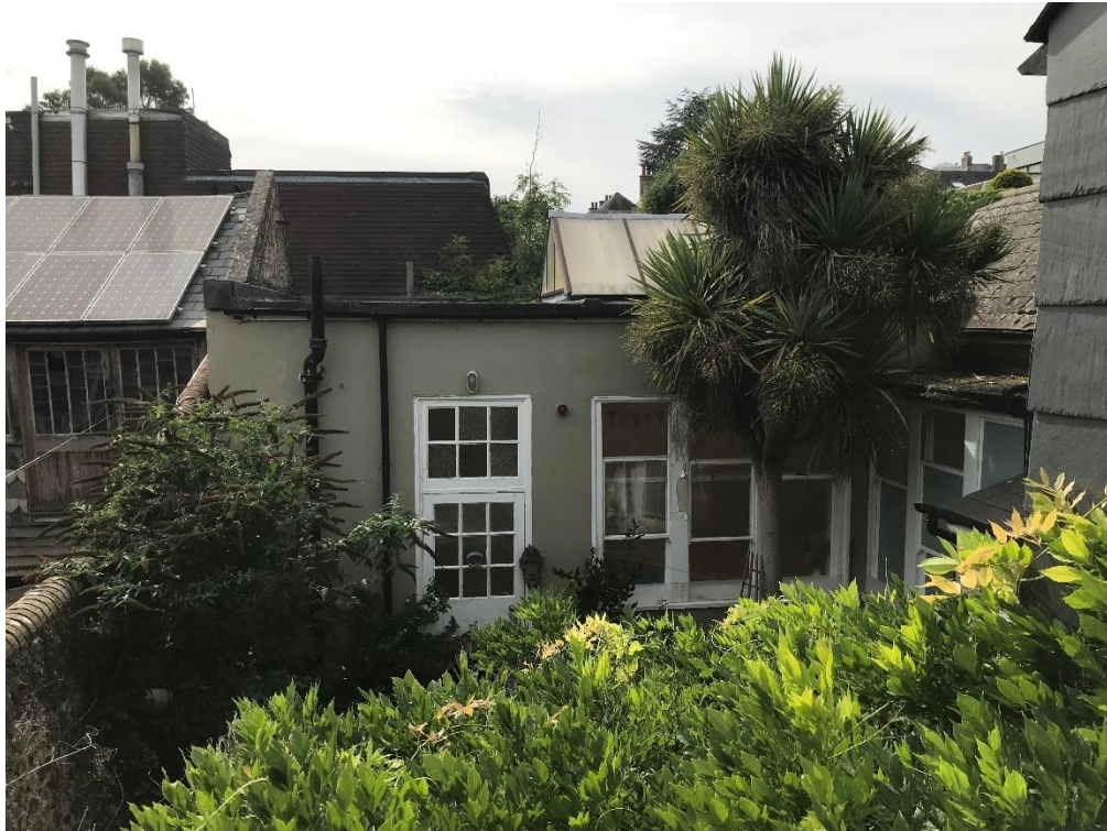
Figure 26: View of the rear part of No. 26A from the garden of No. 26 Station Street.
