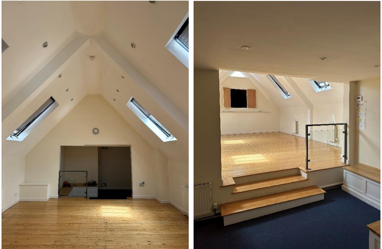
Figure 18: Post 2000 era roof extension looking east (left) with modern partitions to form the staircase landing and anteroom, and view west (right).
