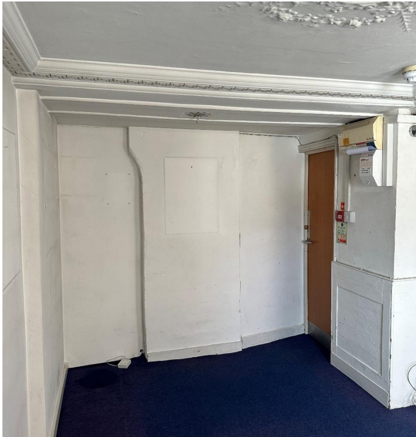
Figure 23: chimney breast to ground floor front room.
