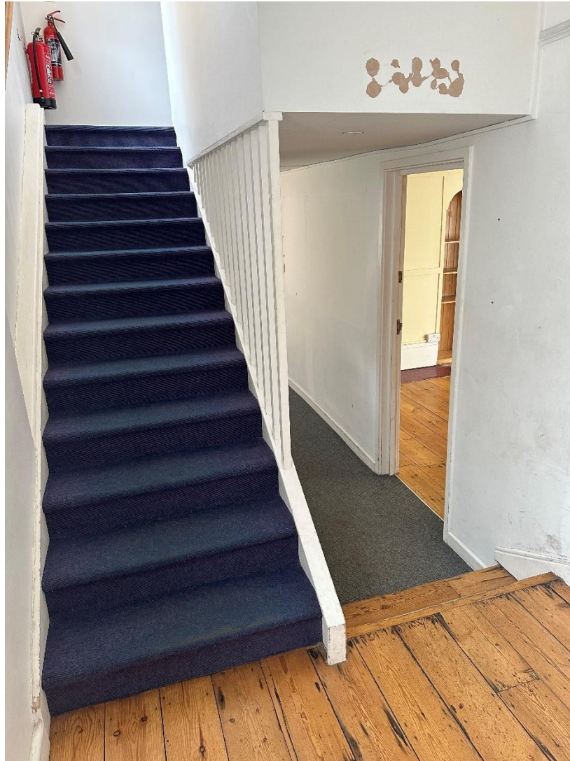
Figure 17: View of ground to first staircase inserted after 2000.
