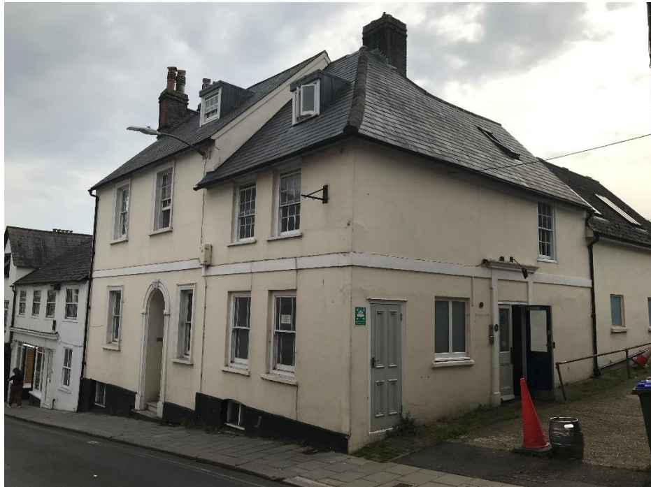
Figure 4: Nos. 26 & 26A Station Street viewed from the north
