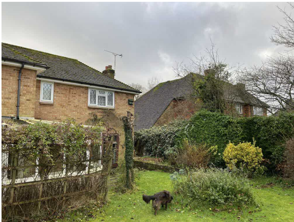
Photograph taken Jan 24 showing the existing rear elevation of 5 Buckmore Avenue and its conservatory. The photograph also shows the side/ rear elevation of the garage to 7 Buckmore Avenue
