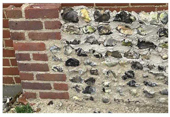
When excavating the footings for the new wall we have found a fair few tonnes of flint from the original wall and are reusing as much flint as possible.
