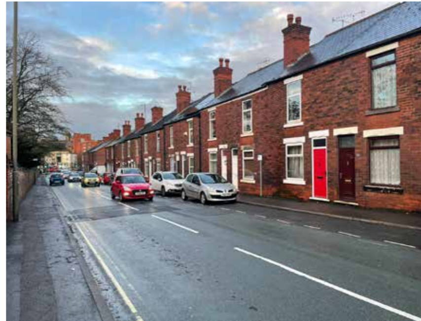
Rows of Red brick Terraced houses along Park Road
