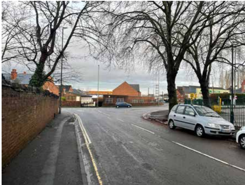
Photograph illustrating highlevel boundary wall that runs along the perimeter of Queens Park abutting Park Road and Boythorpe Avenue.
