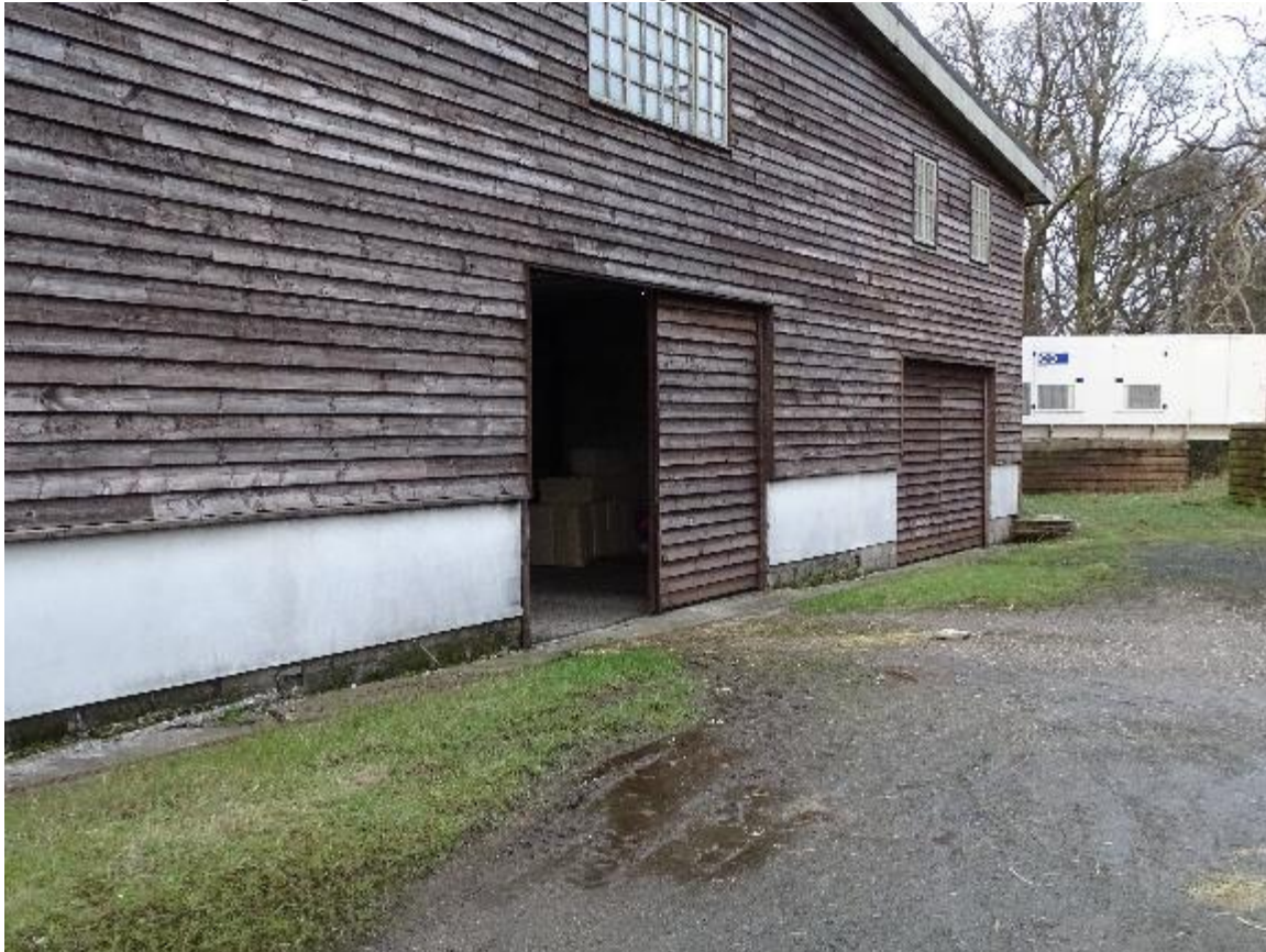
Eastern boundary, inc generator to rear of building One
