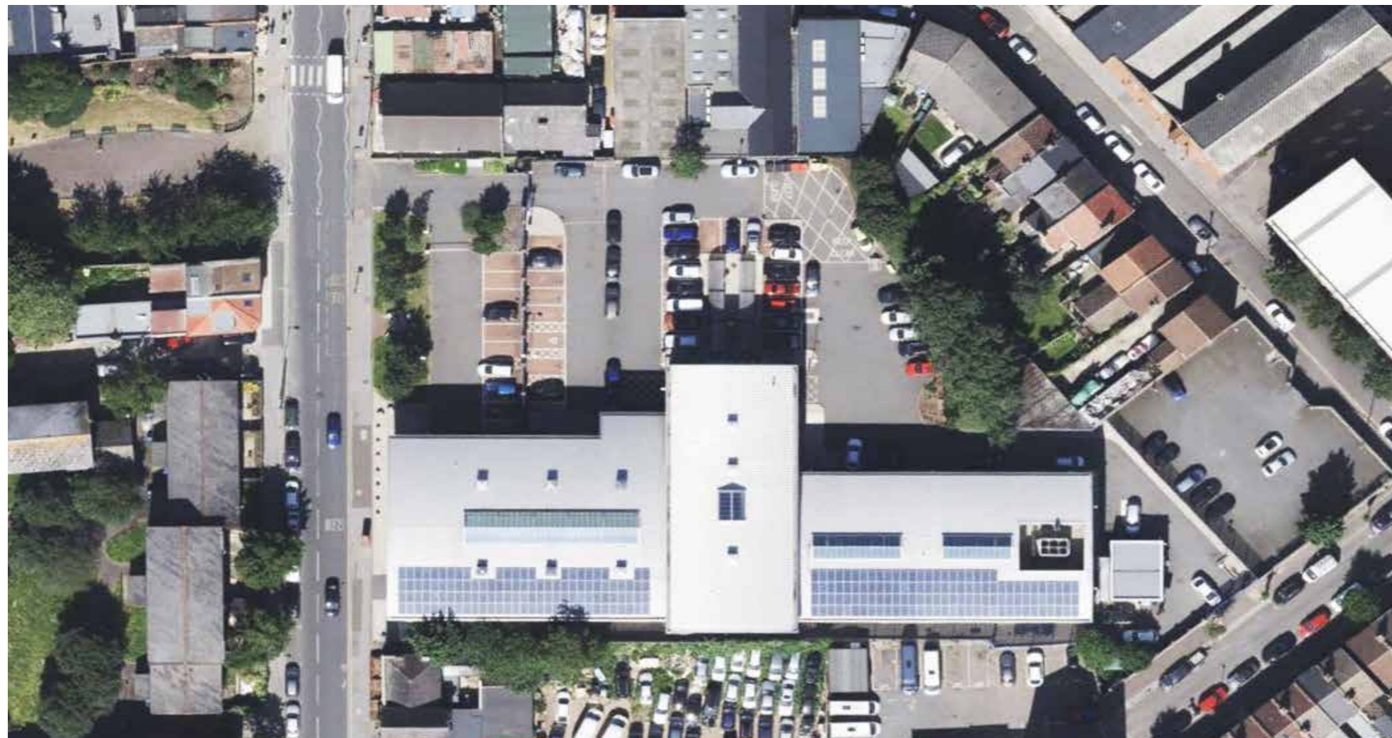
Existing aerial view of site showing roof and car park and service yard beside building.
