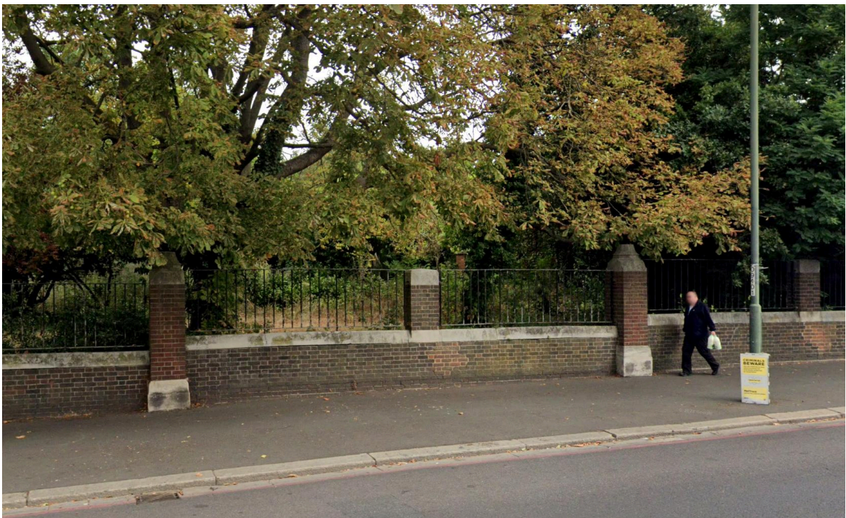
View of the boundary wall to be altered.
