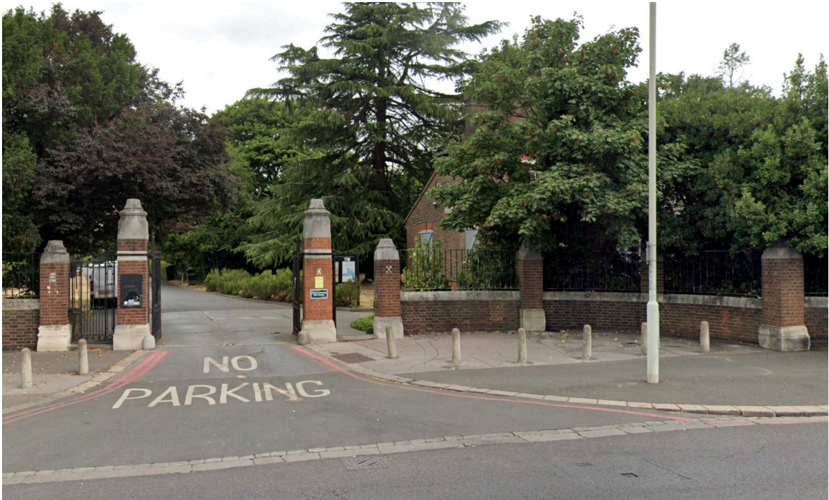
View of the existing Cemetery Gate along Thornton Road
