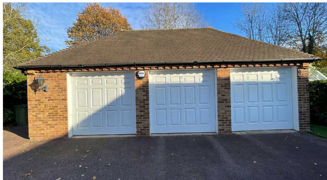
Fig.5 - Existing garage to be demolished
