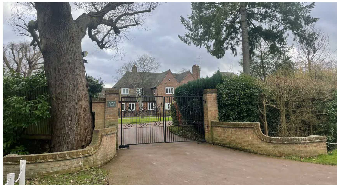
Fig.3 - Existing site entrance from Langworthy Lane
