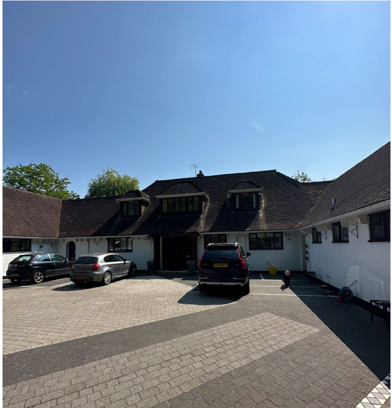
Figure 3 - Existing Residential Dwelling at the Site – Front and Rear Elevations
