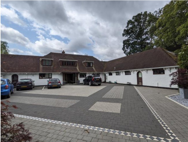
Photo 1: Looking at main house across paved driveway.
