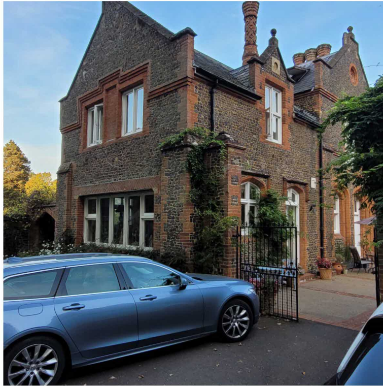
Fig. 2 South west corner of 16 Albury Park Mews
