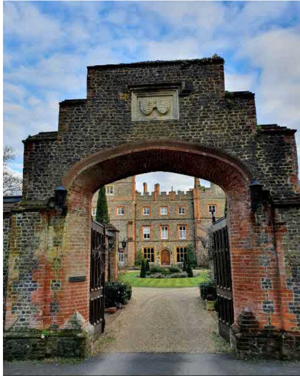
Fig. 10 Photograph of listed Entrance and Walls courtesy of Charles Jennings, dated 10 March 2021
