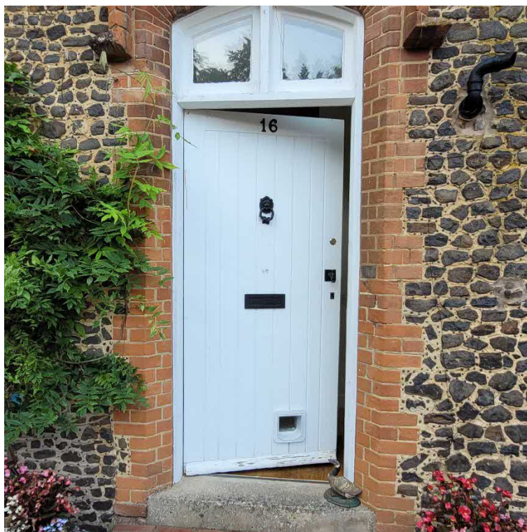
Fig. 5 Photograph of entrance door (South elevation)
