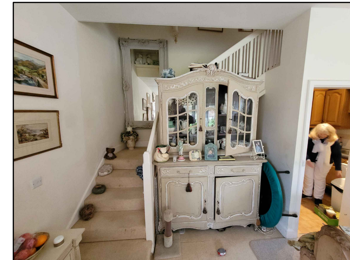
Existing Image of the Stairs
