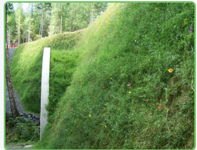
10m (33ft) tall municipal roadway
