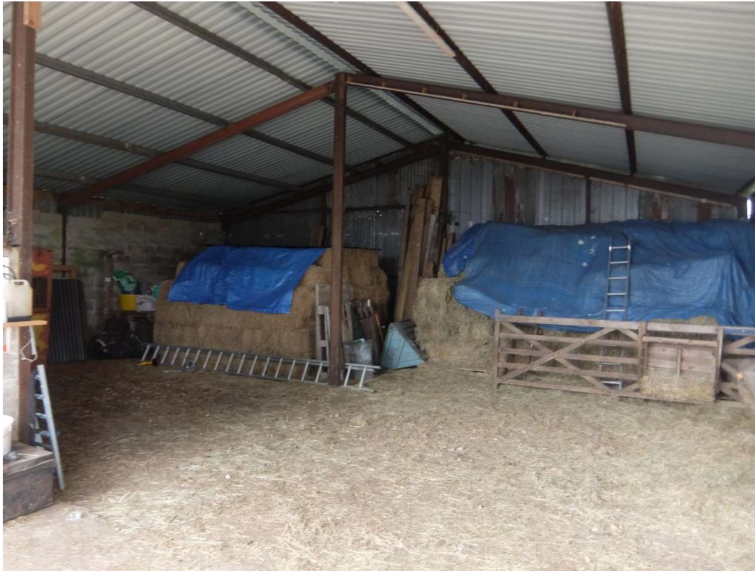
Internal view looking towards rear gable wall
