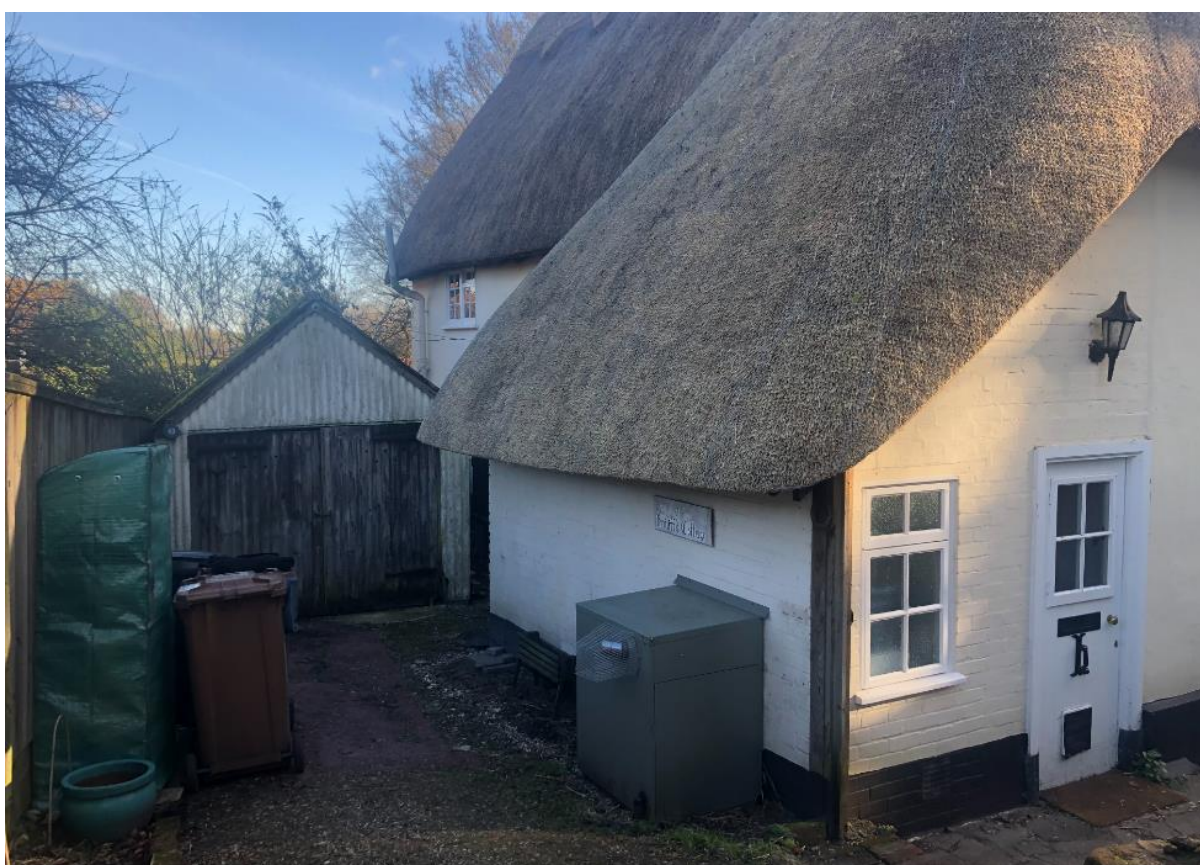
Figure 7 - Photograph of the rear elevation showing the existing garage in situ
