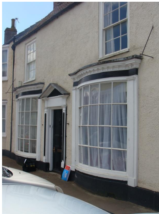
Above: image showing the existing windows 1 and 2.
