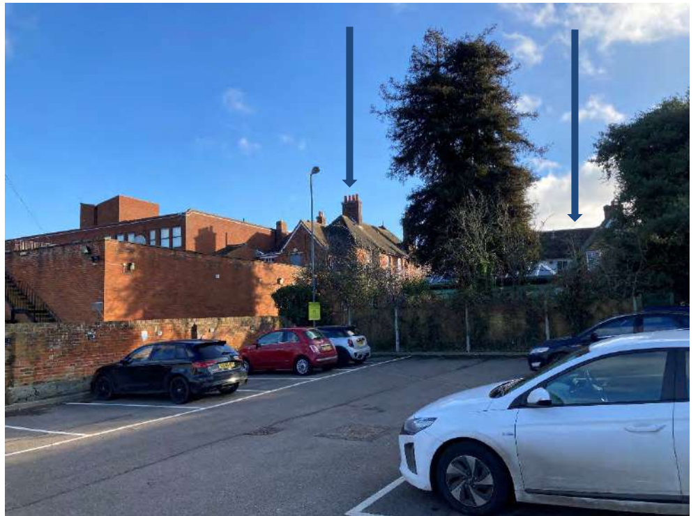
Plate 3 View north-east showing the rear (north-west) elevations 89 High Street (left arrow) and the Grade II listed 'Offices of North Thames Gas Board' (right arrow) which can be glimpsed through the existing vegetation. Note this view is taken from the existing car park which is included within the site boundary. This private parking area is to be retained as part of the proposals.
