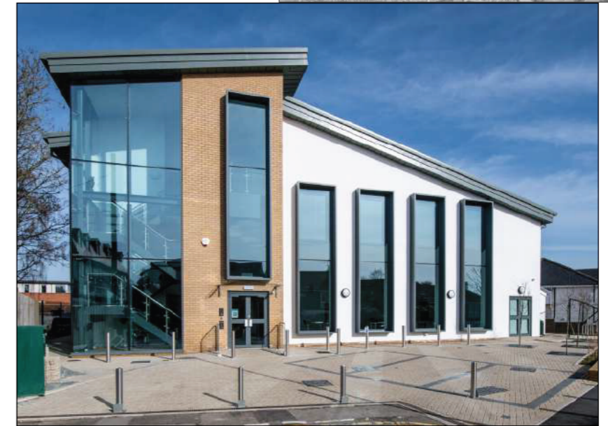
3 CHANTRY CENTRE AND TOWN COUNCIL
