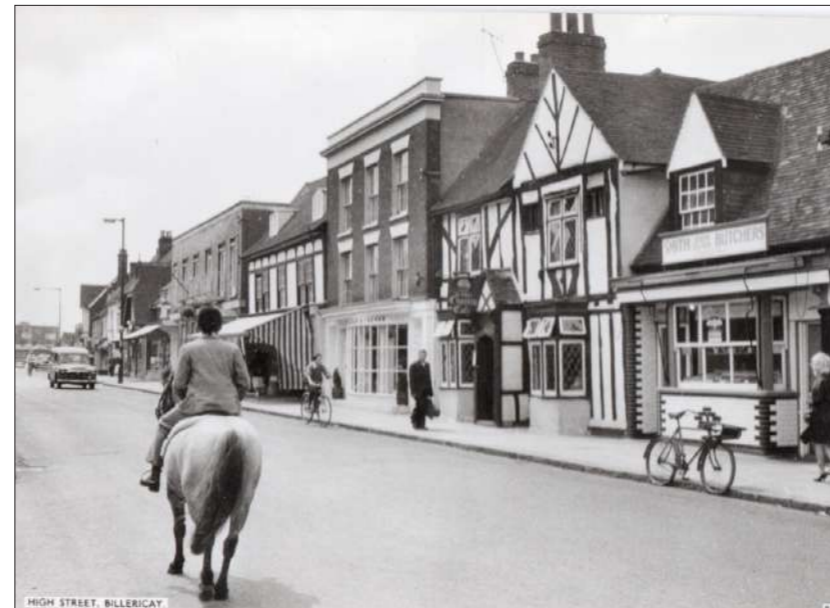
Chantry House, c.1960
