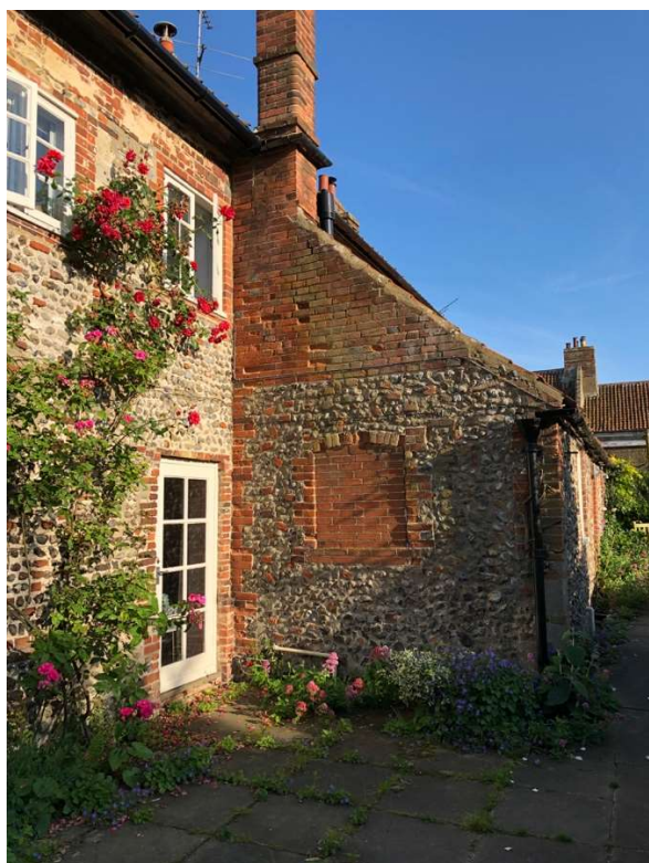
the bricked up window in the west extension
