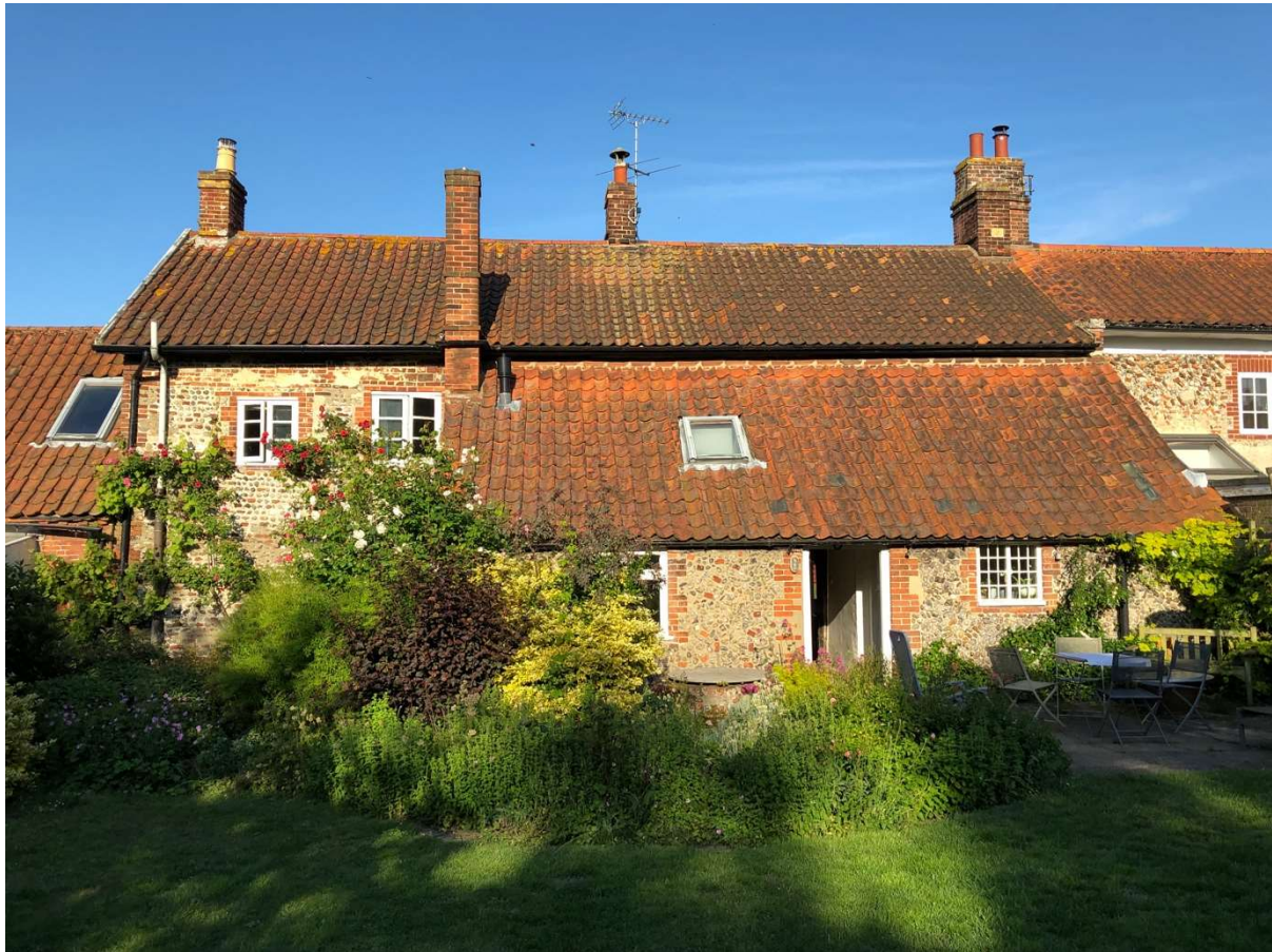
the west garden elevation of the original house and west extension
