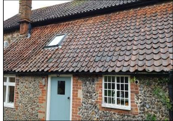
Figure 2: Western aspect extension.
