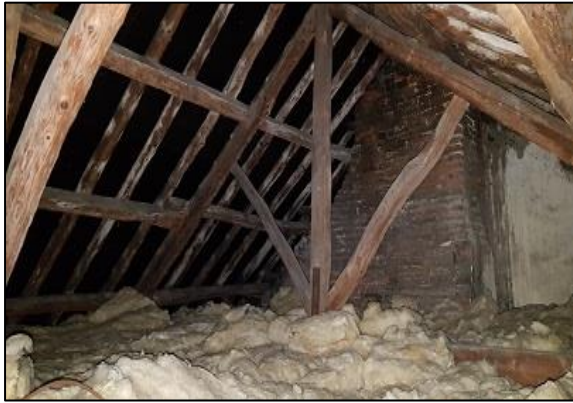
Figure 7: Internal view of main house roof void.
