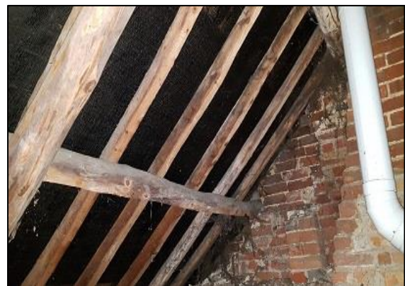
Figure 10: Western extension roof void.
