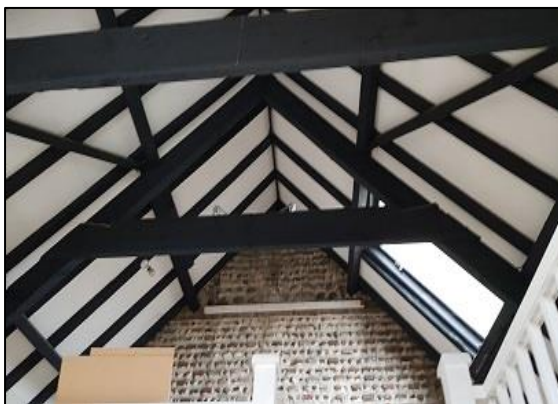
Figure 9: Internal view of northern wing.
