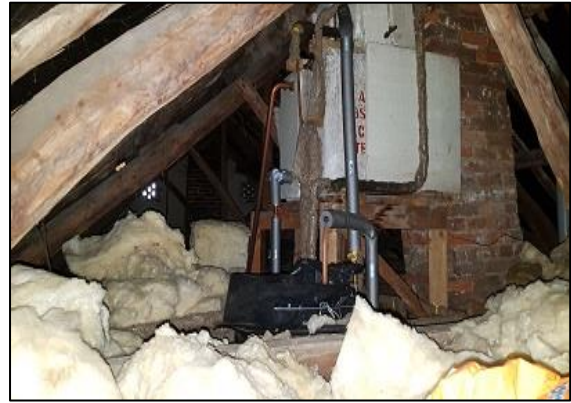
Figure 8: Internal view of main house roof void.
