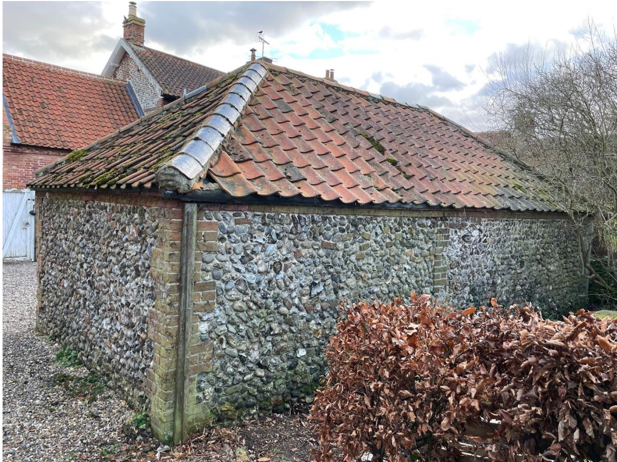
The rear wall of the Cart Shed facing the garden
