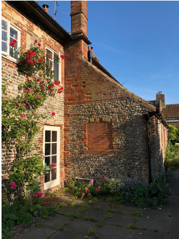
the bricked-up window in the west extension
