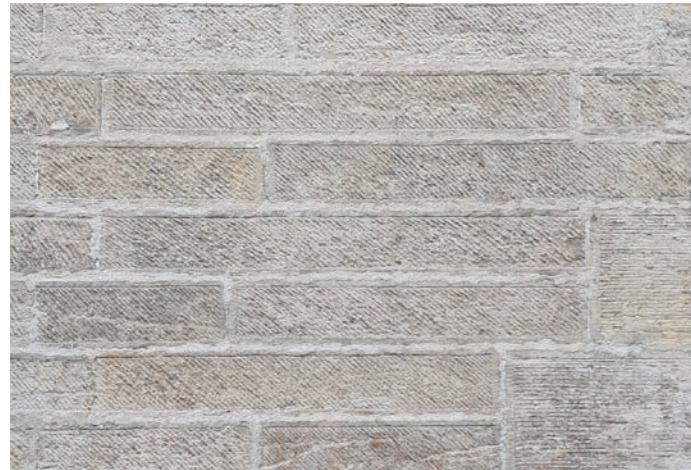
1 - Light grey sandstone with textured angle droving marks
