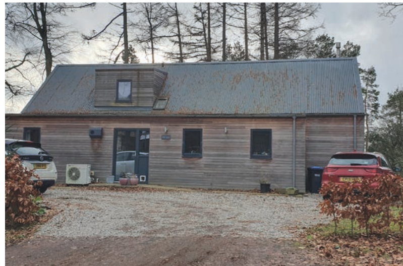
Contemporary new build off Medwyn Road
