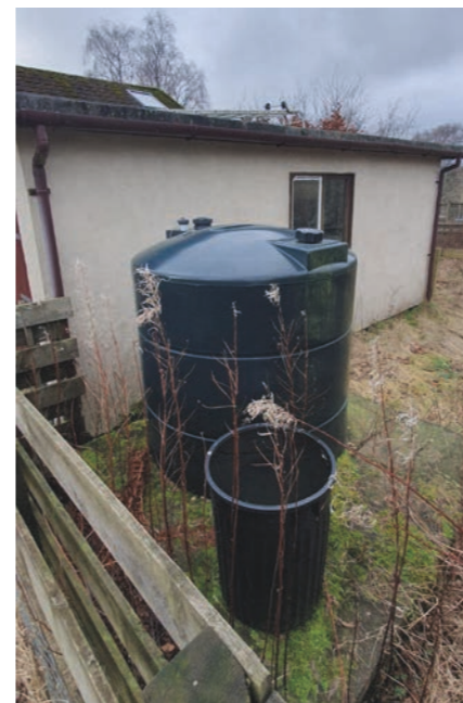
Existing oil tank
