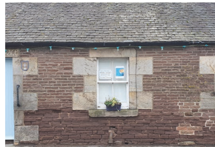
9 - Rich red sandstone with brick scale regular coursing, rybat contrast
